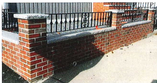
Decorative Metall Railing Mounted to Brick Veneer Wall
