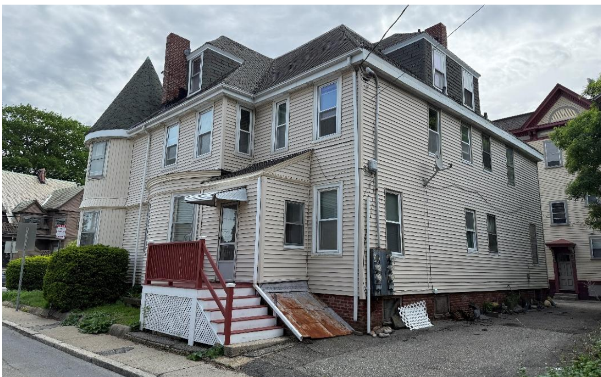
178-180 Elm Street North, west (side) and rear elevations
