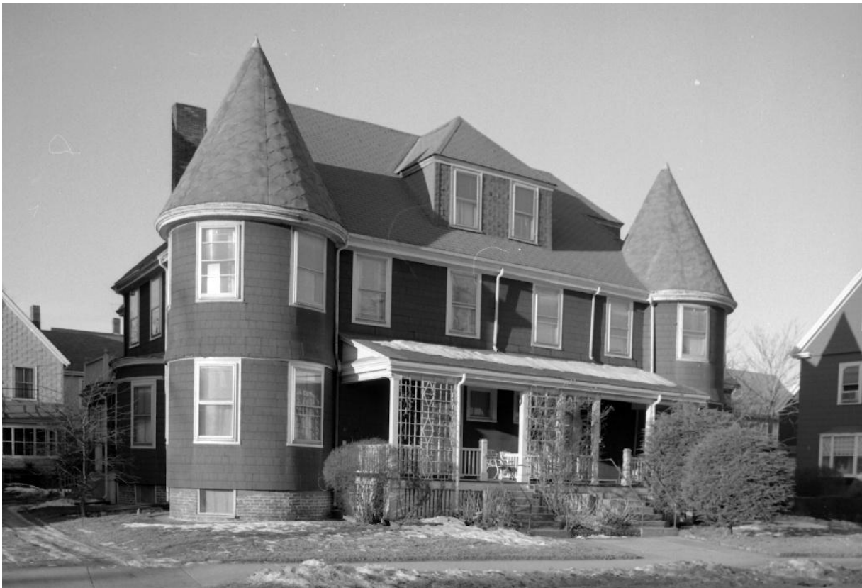
178-180 Elm Street North
