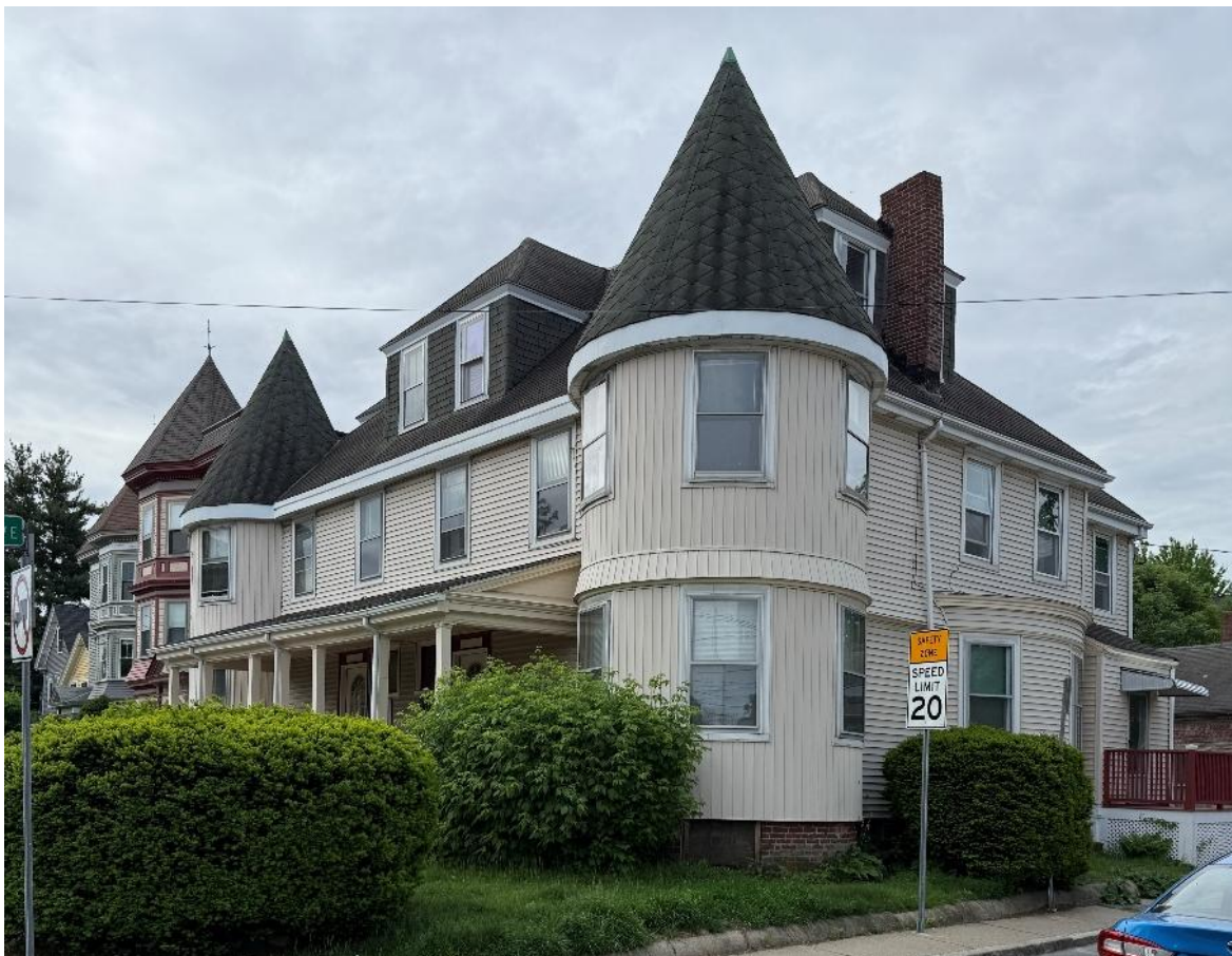
178-180 Elm Street North
