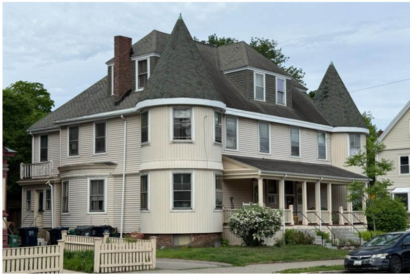
178-180 Elm Street North
