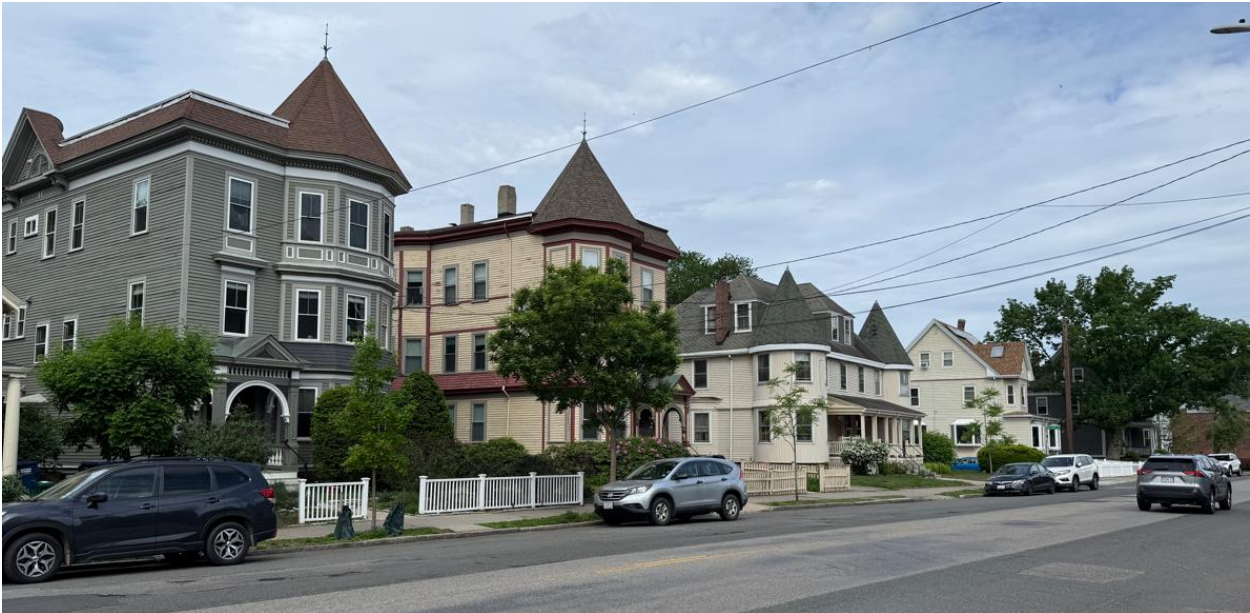
Elm Street N Streetscape. L-R: 174 and 176 Elm (both 1892), 178-180 (1892), and 182 (1894) CHC, 2026
