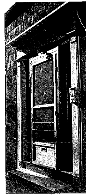
173. Front entrance, 98 Spring Street, 1840. Photograph 1964 O
