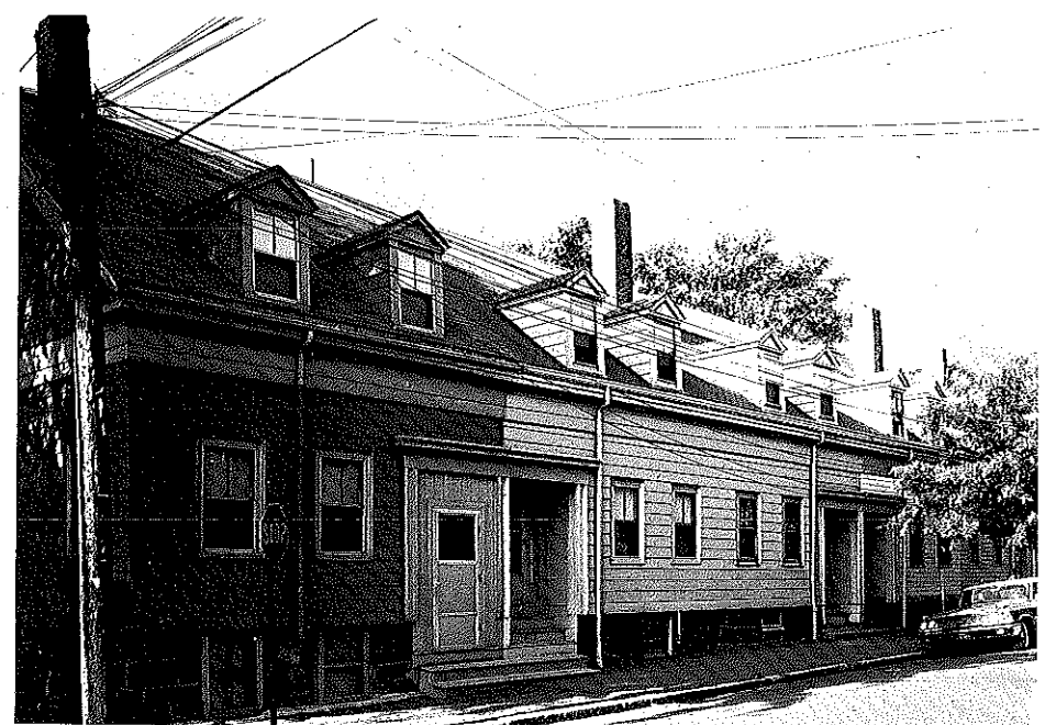
213. 84-92 Spring Street, 1844. Photograph 1964
