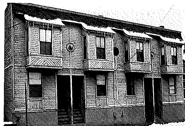
250. 53-59 Sciarappa Street, 1882. Photograph 1964
