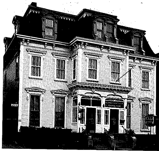
243. 390-392 Cambridge Street, 1869. Photograph 1964
