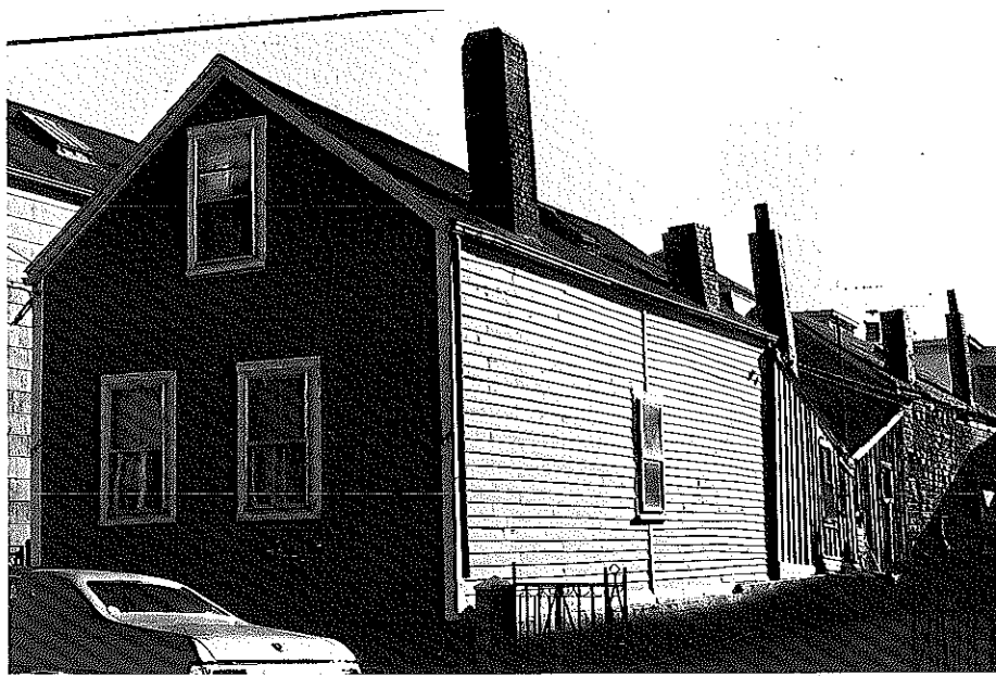
172. Rear facade, 146 Thorndike Street. Photograph 1985 126925/14
