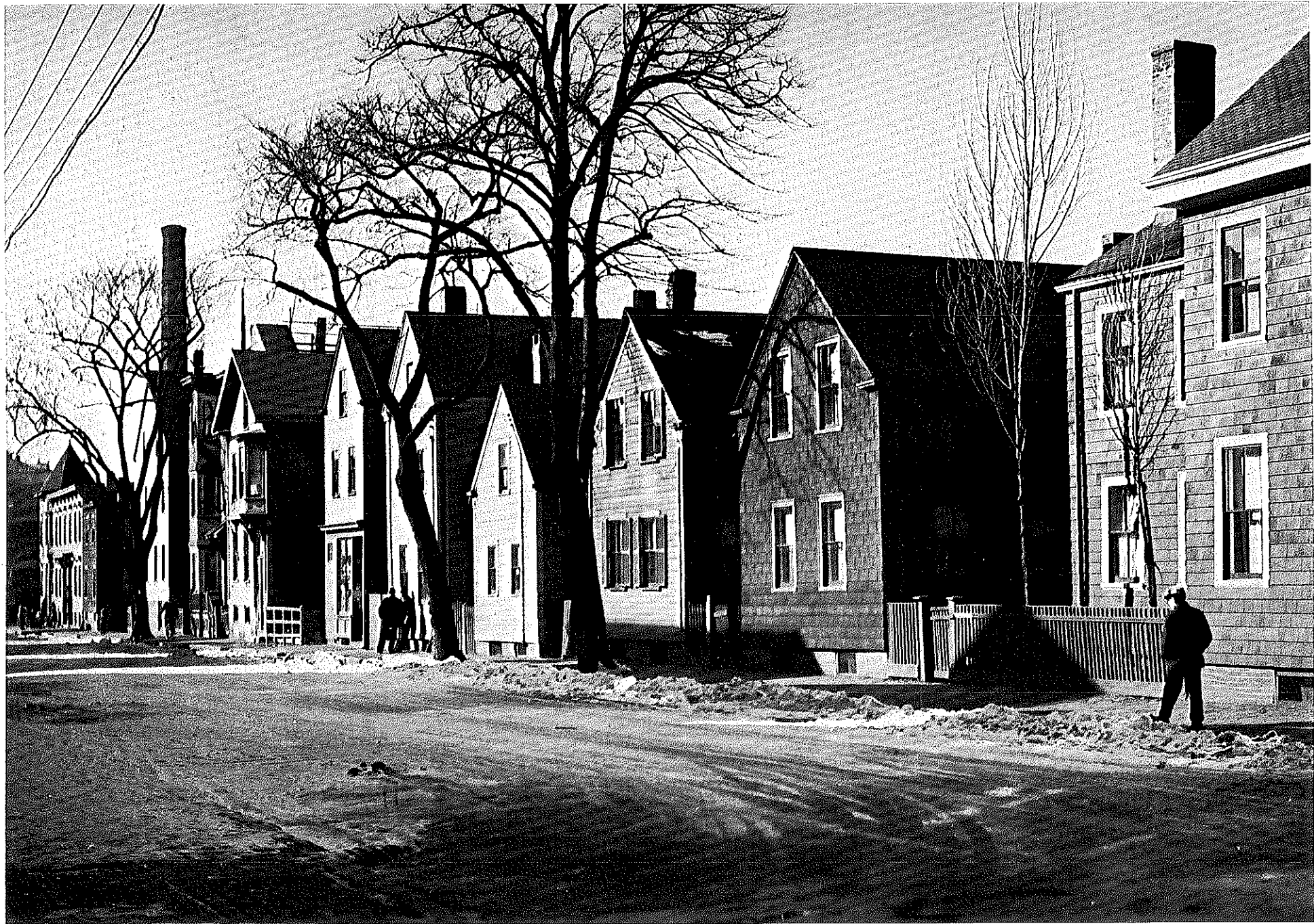
167. Winter Street worker's cottages, c. 1940 missing
