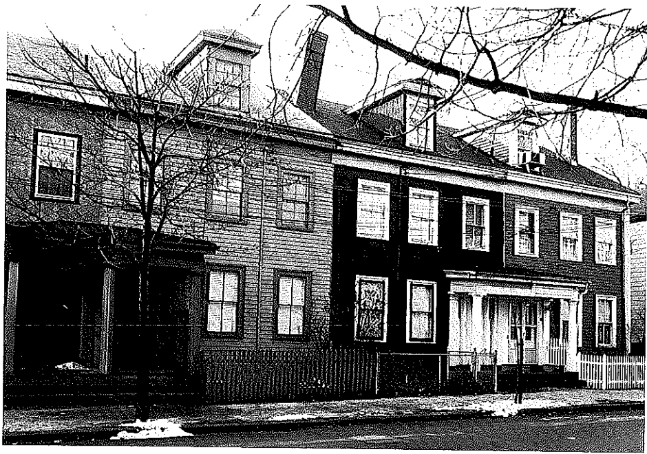
212. 72-78 Spring Street, 1845. Photograph 1964
