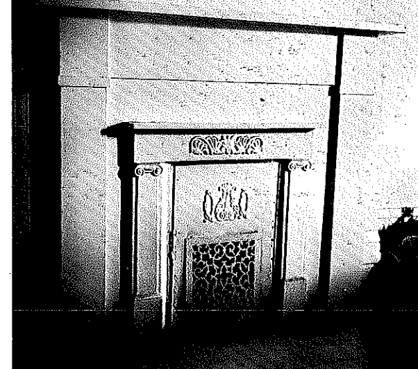
219. Second floor fireplace with hot air register insert, 67-69 Otis Street, 1839 1218/9A
