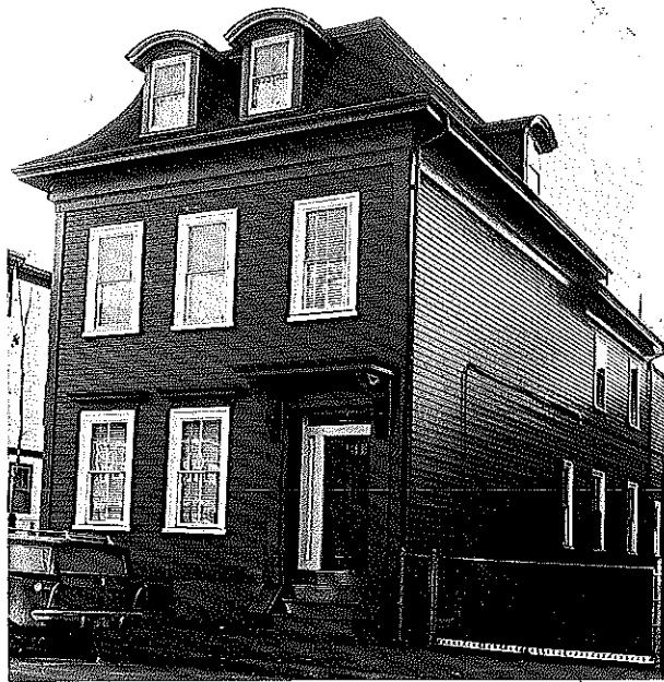
246. 462 Cambridge Street, 1866. Photograph 1964
