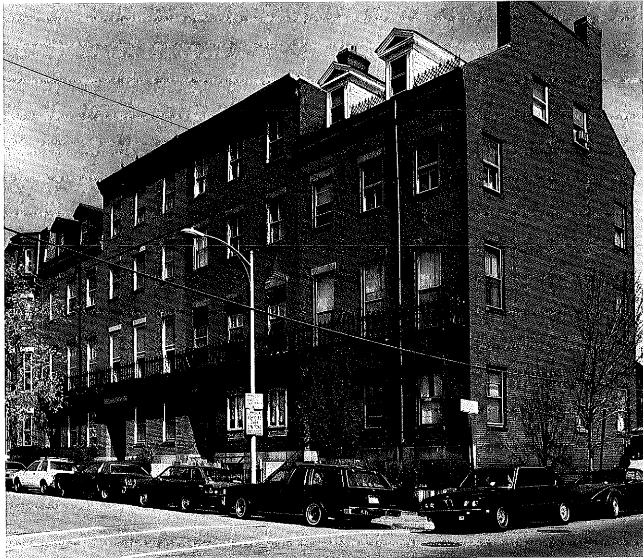
209. 55-61 Otis Street, 1851, William A. Hall, builder 48512/2
