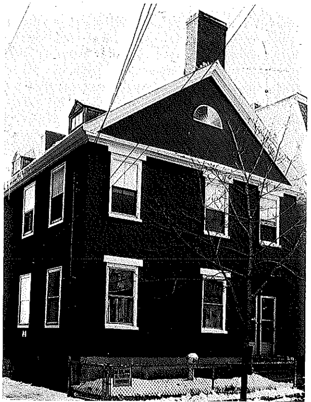
153. 96 Thorndike Street, 1826–27. Photograph c. 1968
