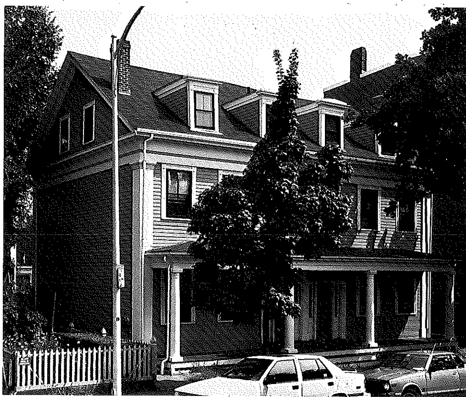
206. 67–69 Otis Street in 1987 (after restoration) ☉
