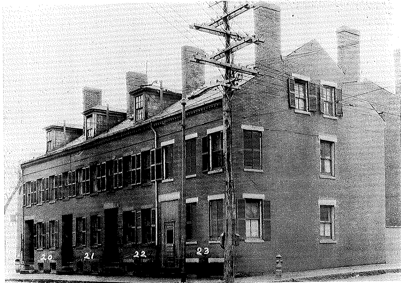
147. Type C row houses, 208-224 Bridge Street, c. 1830. Photograph 1925
