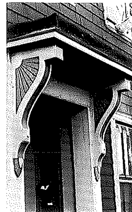
227. Bracketed door hood, added 1880s, 129 Thorndike Street, by 1868 120421/10
