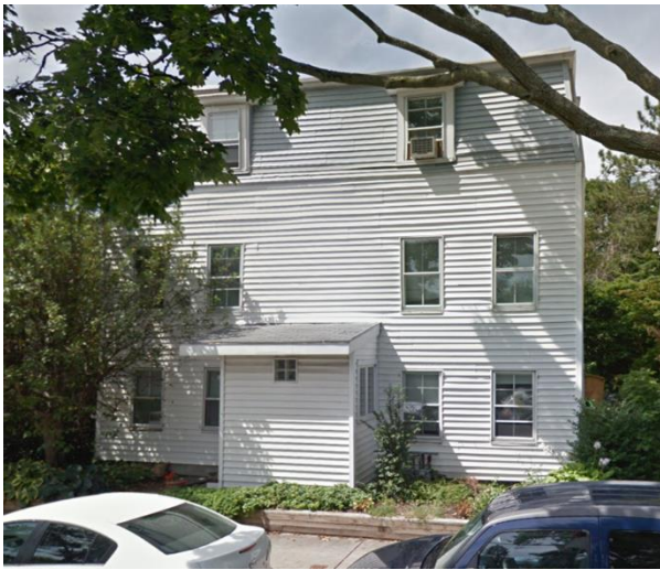
31-33 Willard Street, Before (2011)
