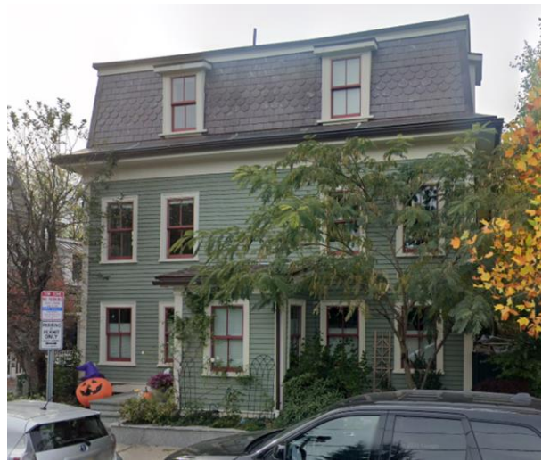
31-33 Willard Street, After (2020)
