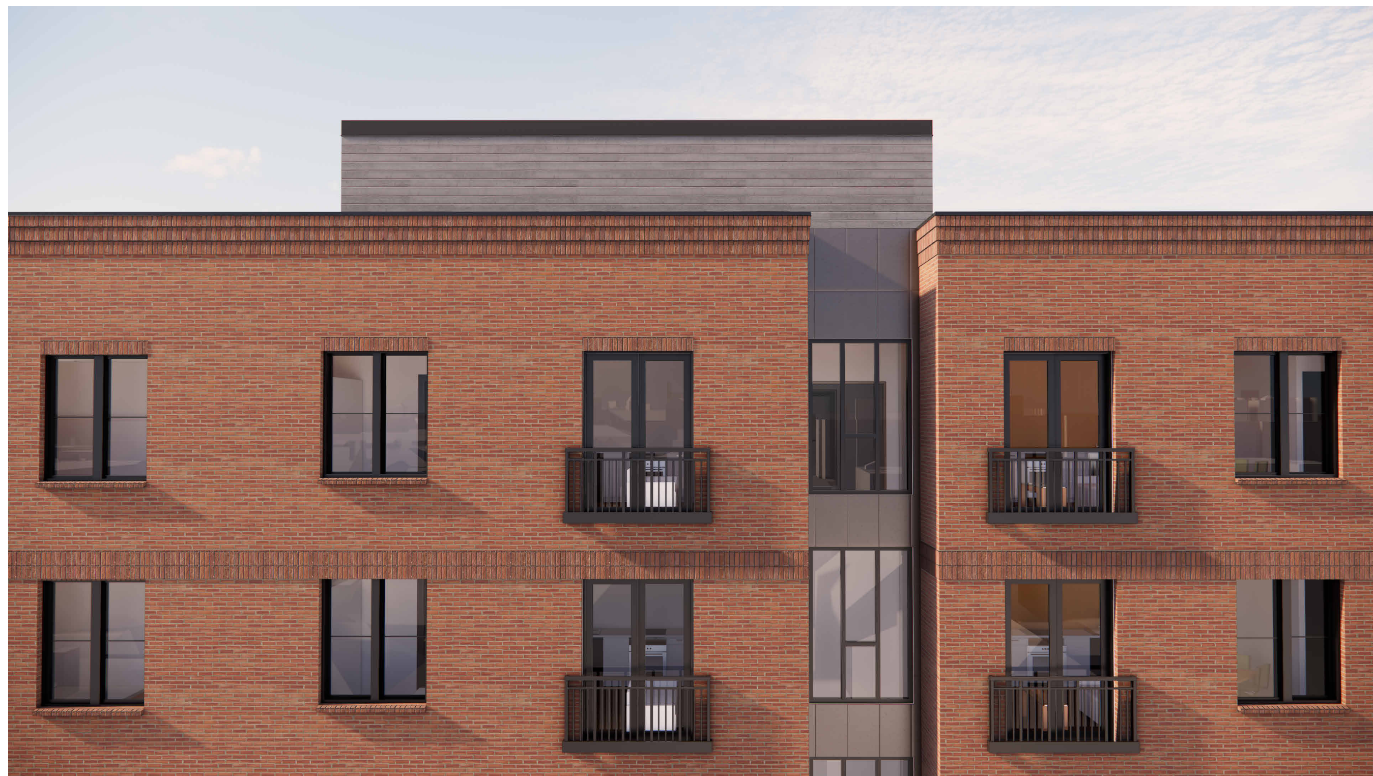
BRICK CORNICE & RECESS DETAIL
