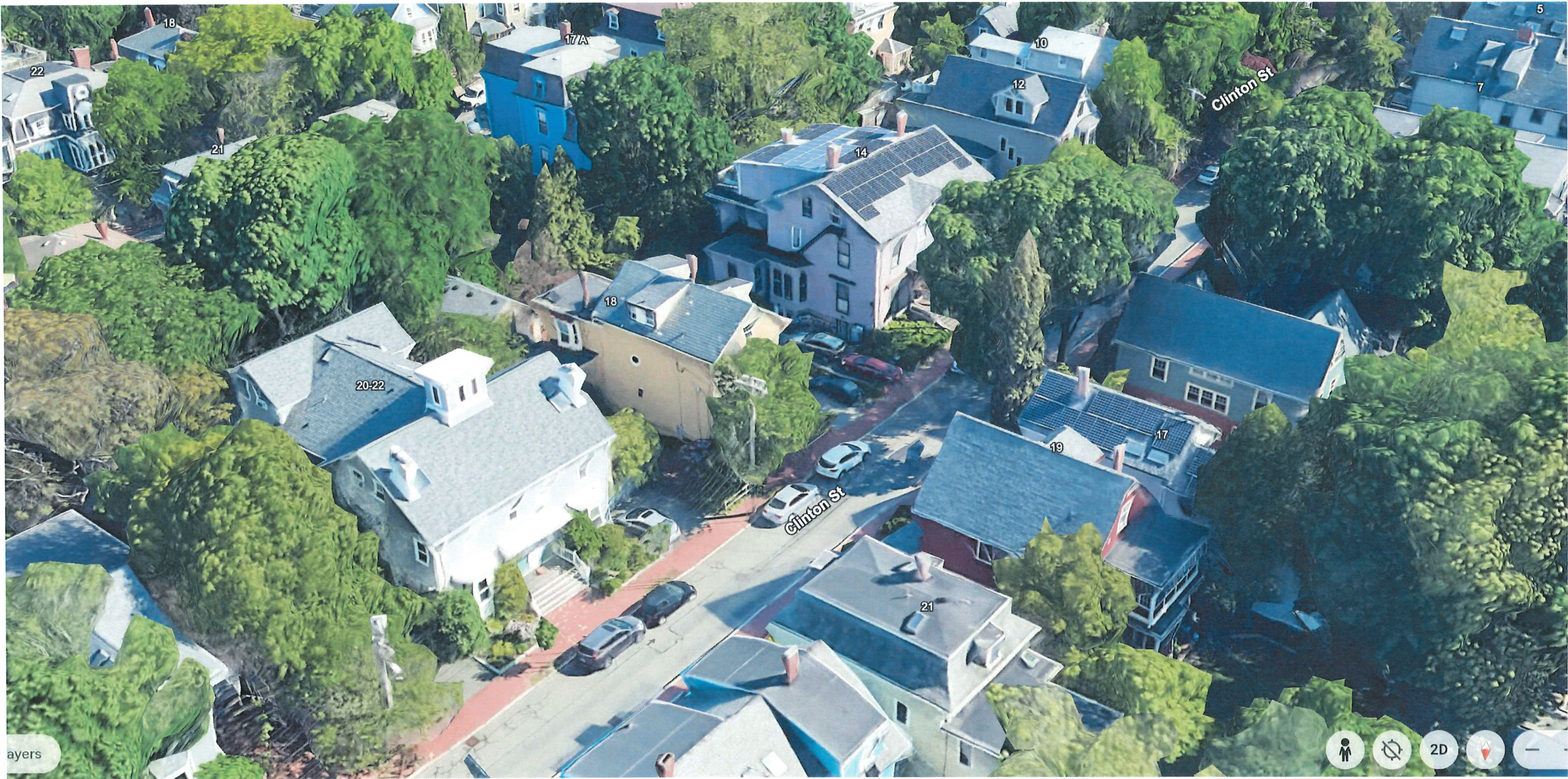
AERIAL VIEW FROM NORTHERN CORNER OF SITE
