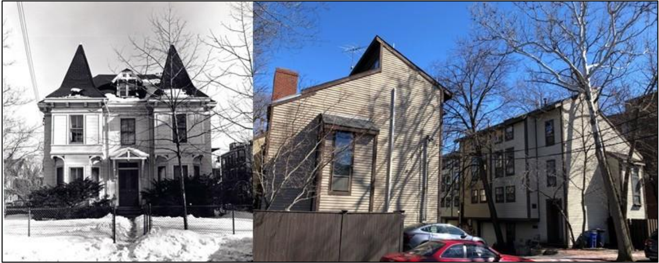
36 Irving Street, 1873 house demolished for the construction of 9 townhouses, 1977.
