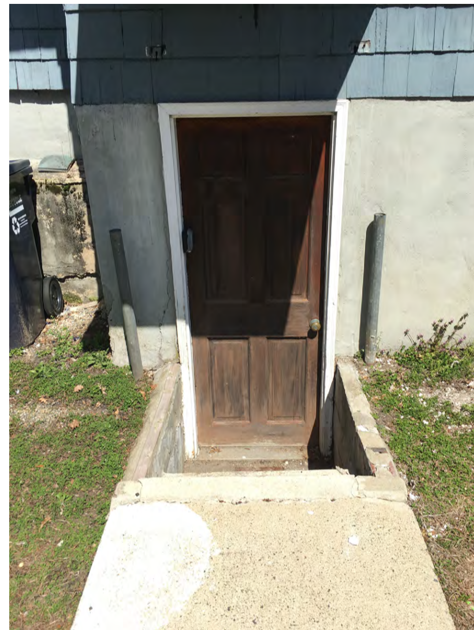
SOUTH - LOWER LEVEL ENTRANCE
