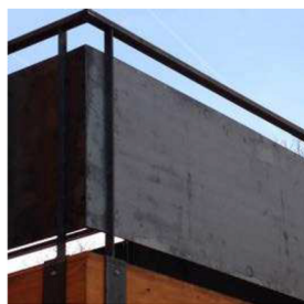
8. Perforated/ Opaque Metal Railing
