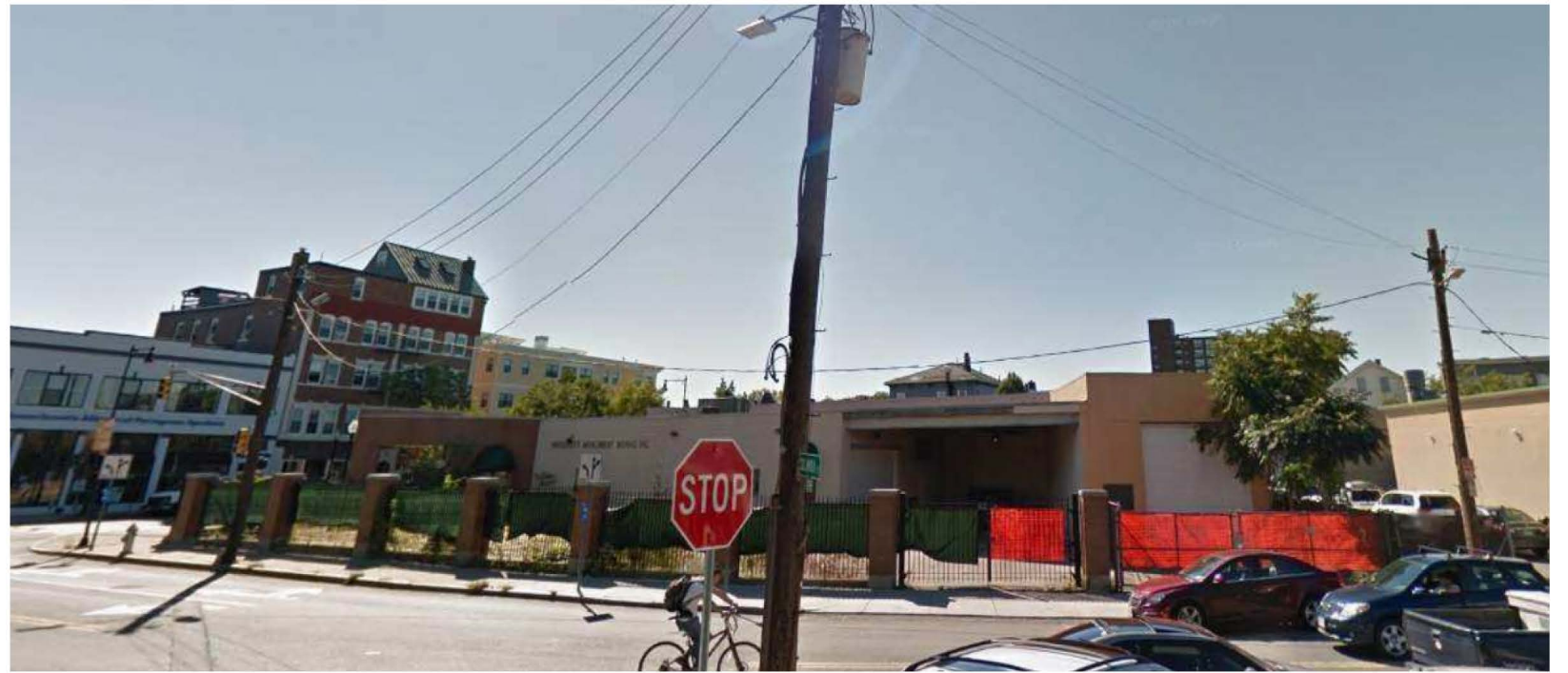
View from Columbia Street
