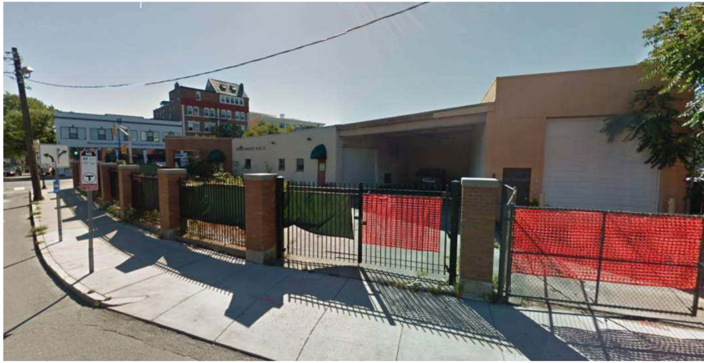
View from Webster Street
