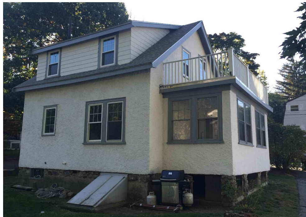
VIEW FROM BACKYARD NORTHWEST
