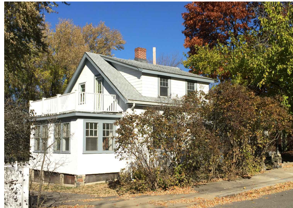
VIEW FROM NORMANDY AVE SOUTHWEST
