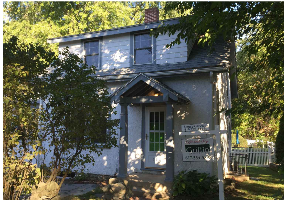
VIEW FROM NORMANDY AVE SOUTH
