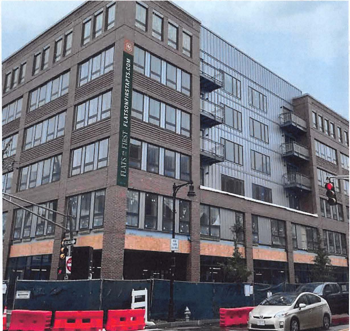
Location 1 - Not Wrapped
