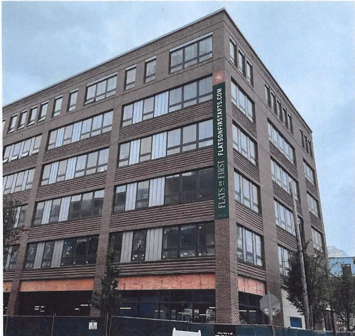
Location 2 - Not Wrapped
