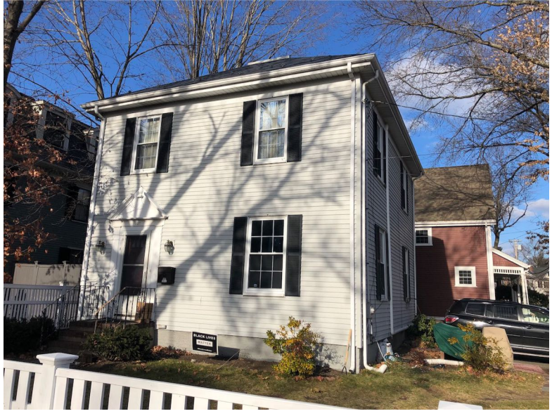
2 Existing Conditions Photograph Scale: None
