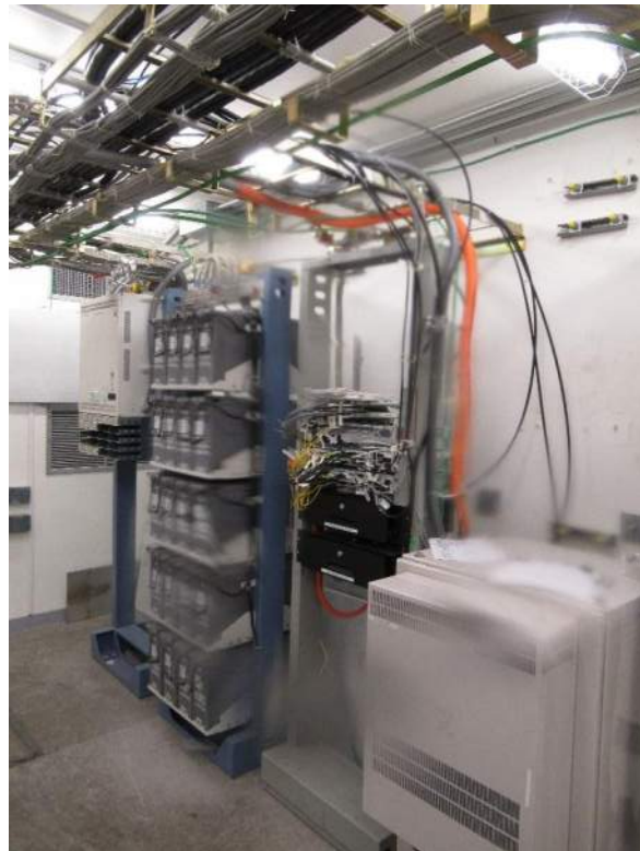
Photo 4: Sample photo illustrating the existing equipment.
