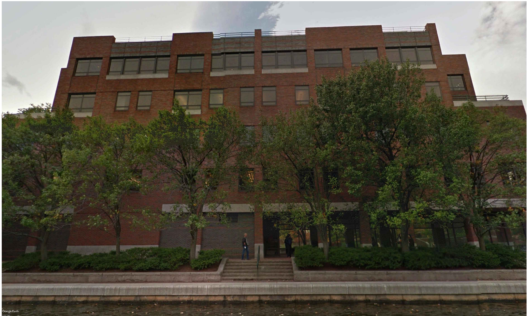
VIEW SOUTHWEST FROM CANAL PARK (EQUIPMENT NOT VISIBLE)
