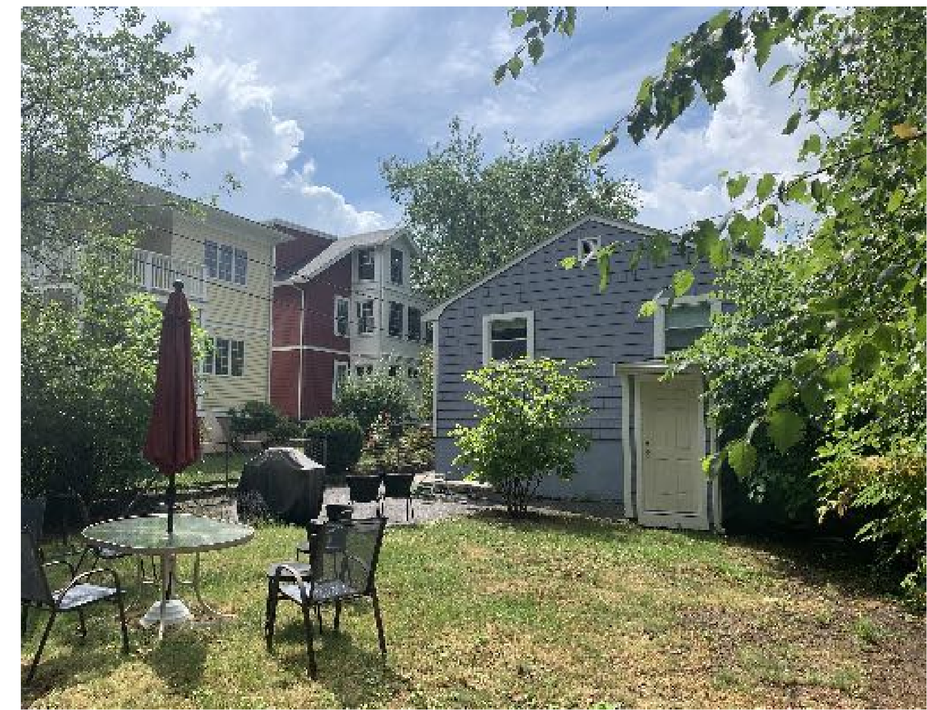
EXISTING REAR FACADE
