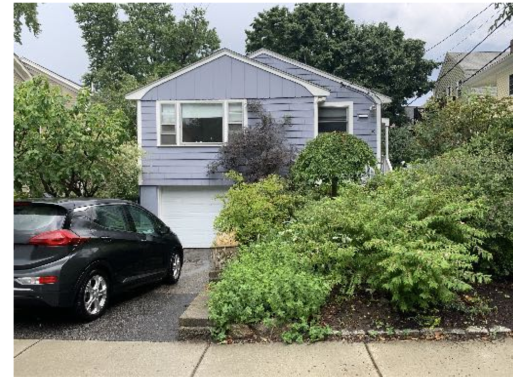
EXISTING FRONT FACADE
