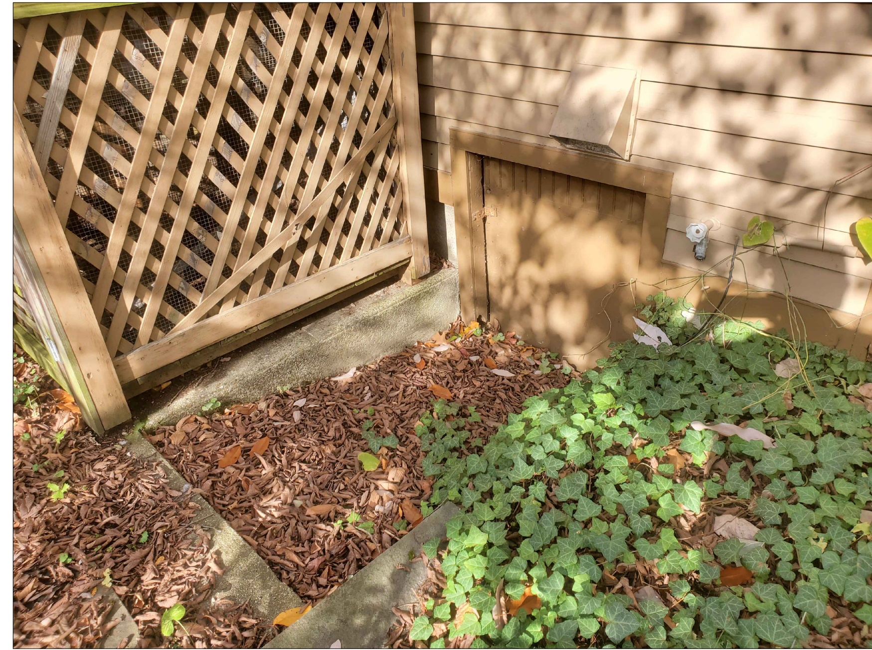
7 Stairs to Crawl Space at South Elevation
