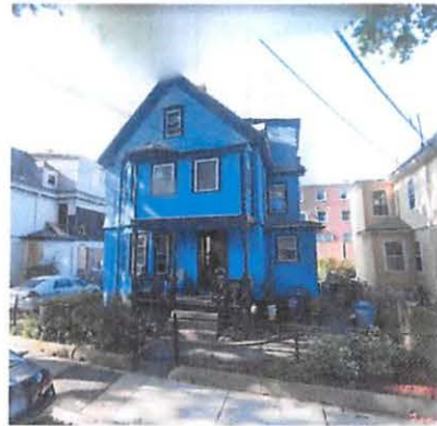
PRIOR TO RENOVATION
