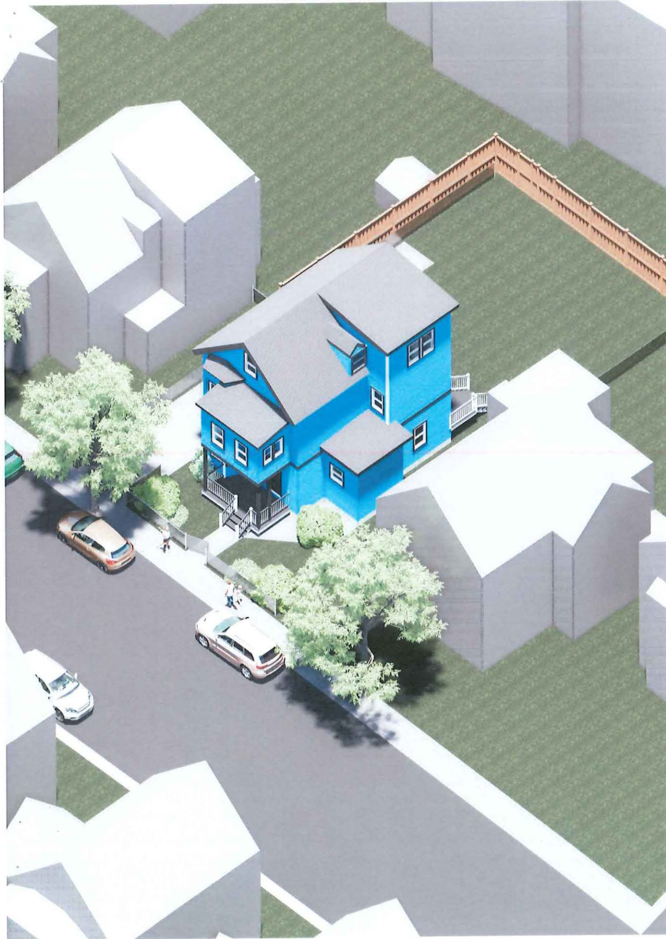
PRIOR TO RENOVATION
