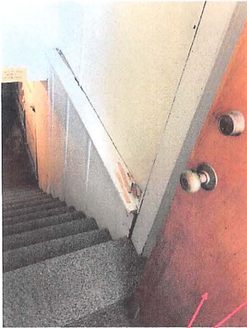
Rear door provides sole access to basement
