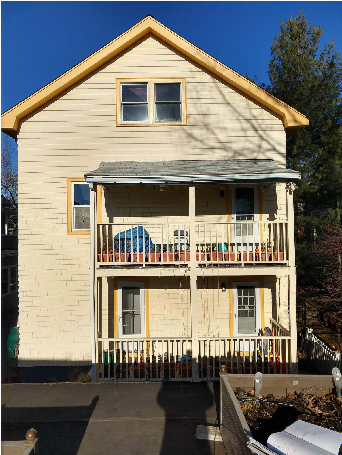
Existing back porch at 116 Henry
