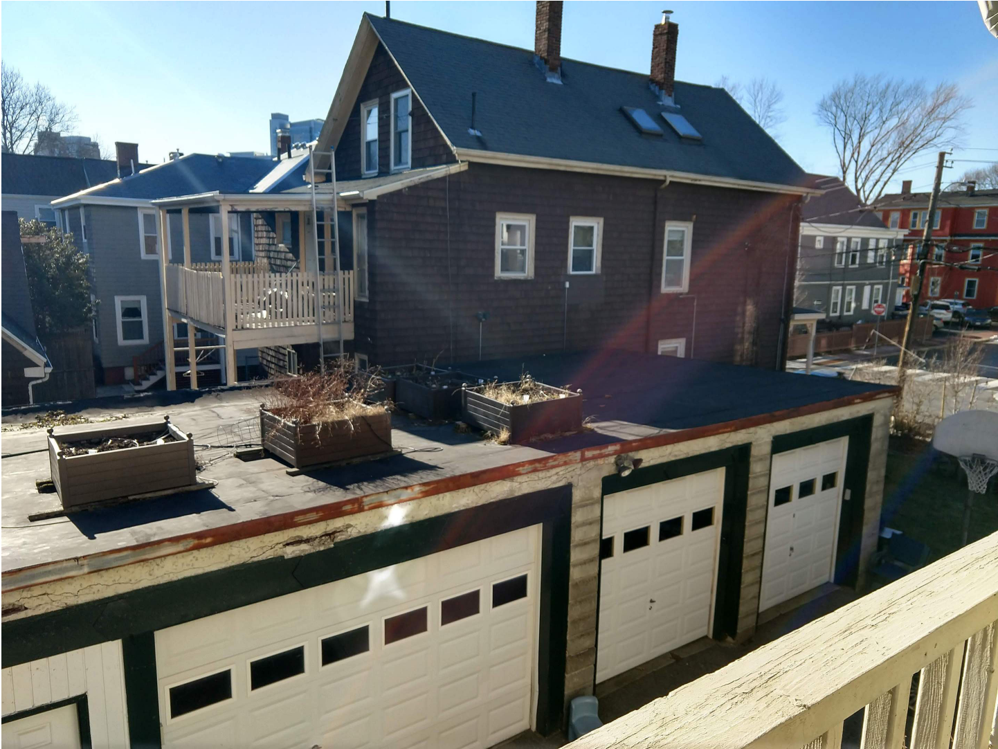
Existing garage roof, 338 Pearl St beyond
