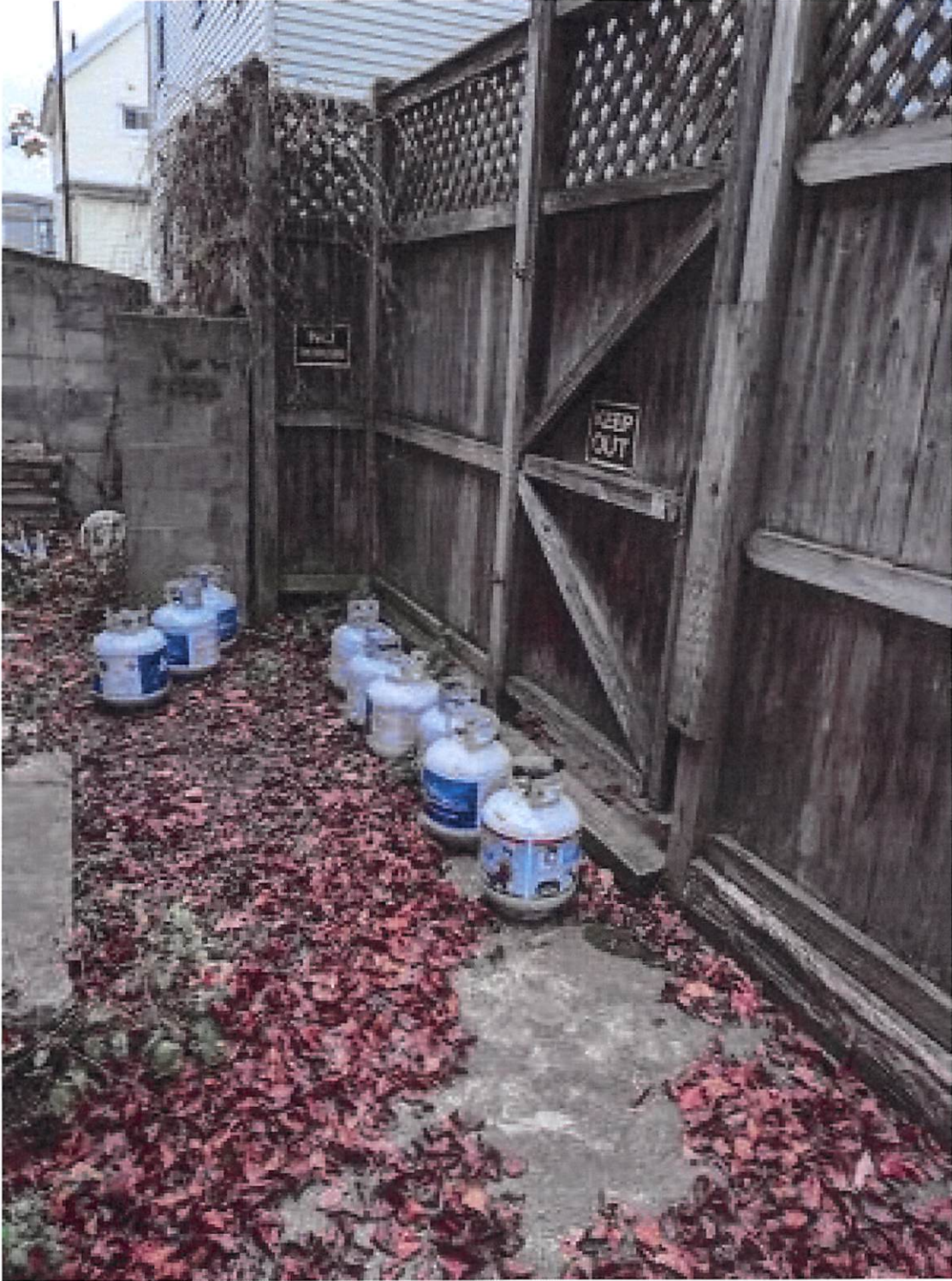
November 20, 2020: use of alleyway to store 9 or more propane gas tanks, including having all of the tanks block the opening of the emergency egress door from the 82-84 Tremont St Condo and creating a fire hazard
