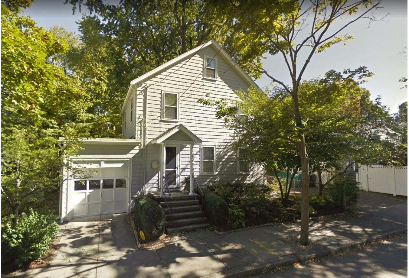
NORTH ELEVATION FROM HUTCHINSON STREET
