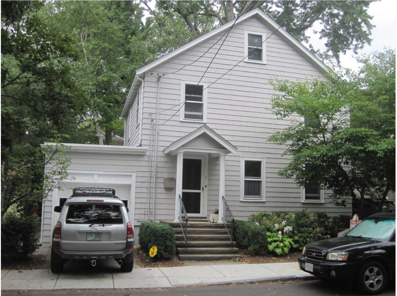
NORTH ELEVATION FROM HUTCHINSON STREET
