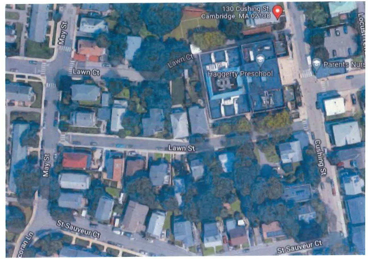
2 AERIAL VIEW GOOGLE MAPS N/S
