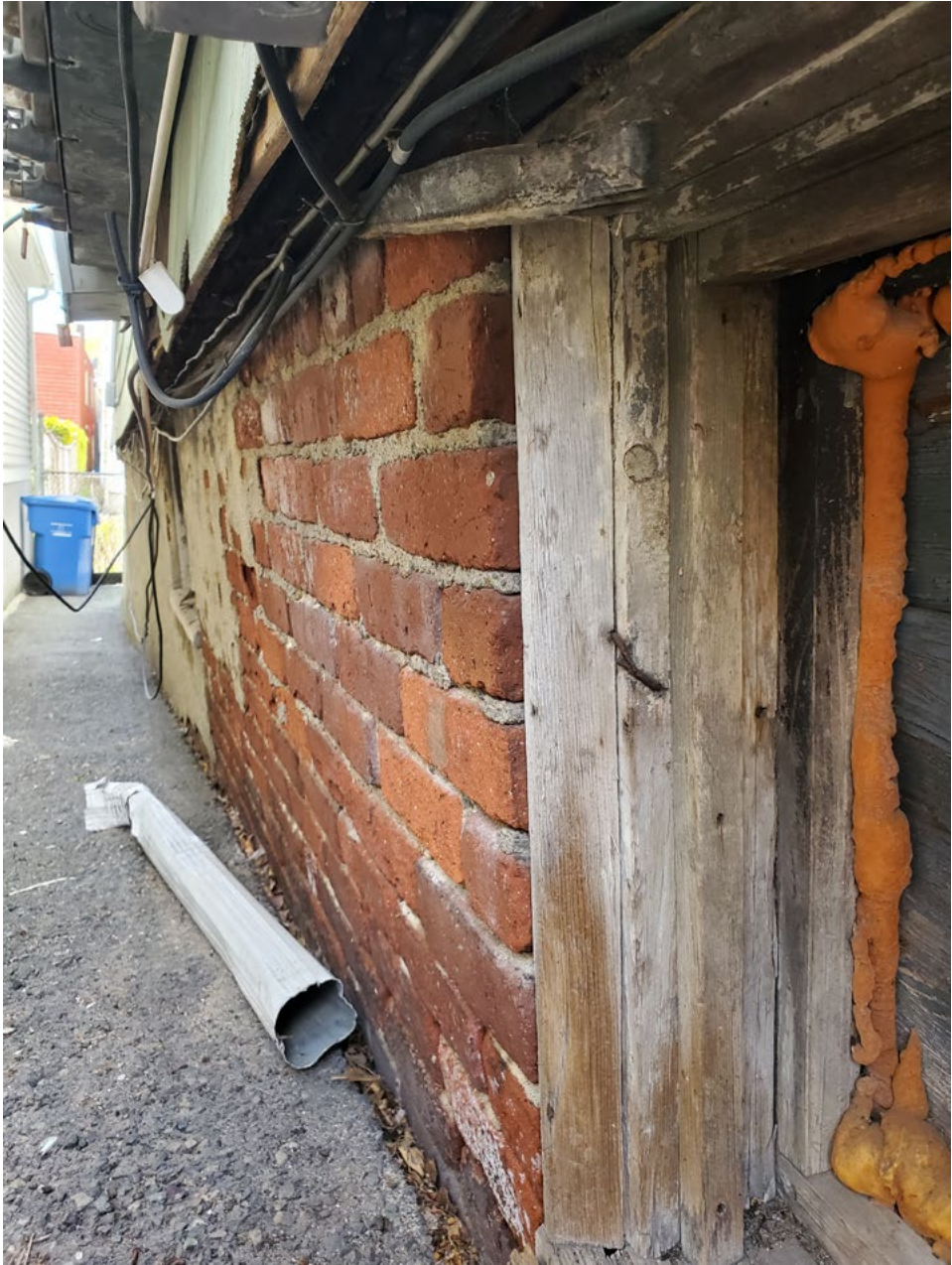
FOUNDATION WALL THAT WILL NEED TO BE FIXED
