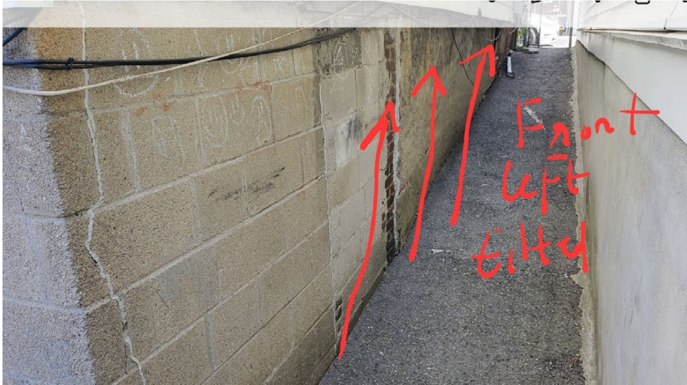
FOUNDATION WALL THAT WILL NEED TO BE FIXED
