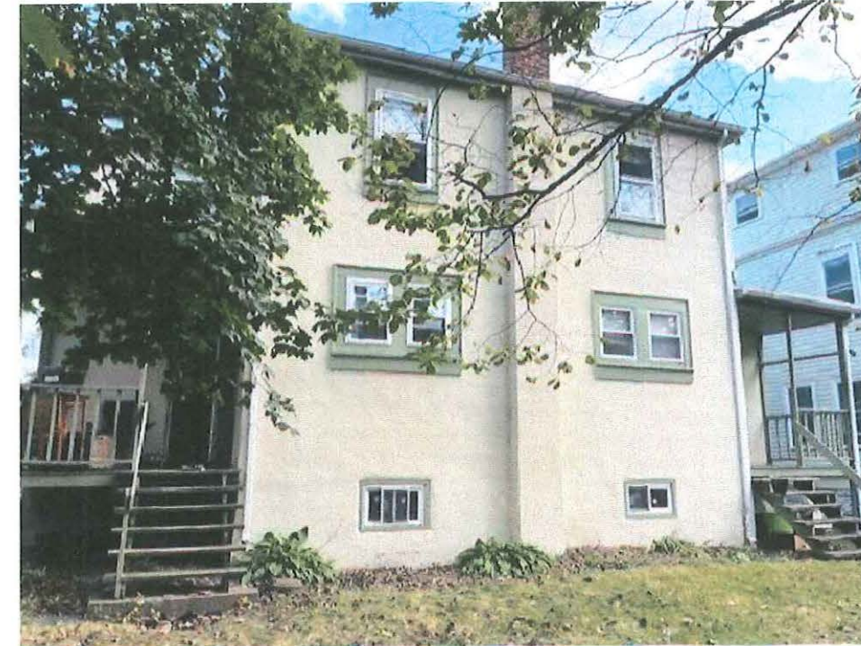
VIEW OF REAR
