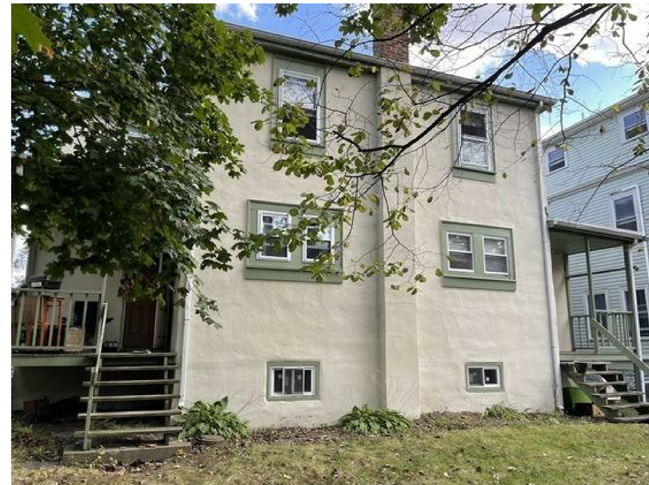
VIEW OF REAR
