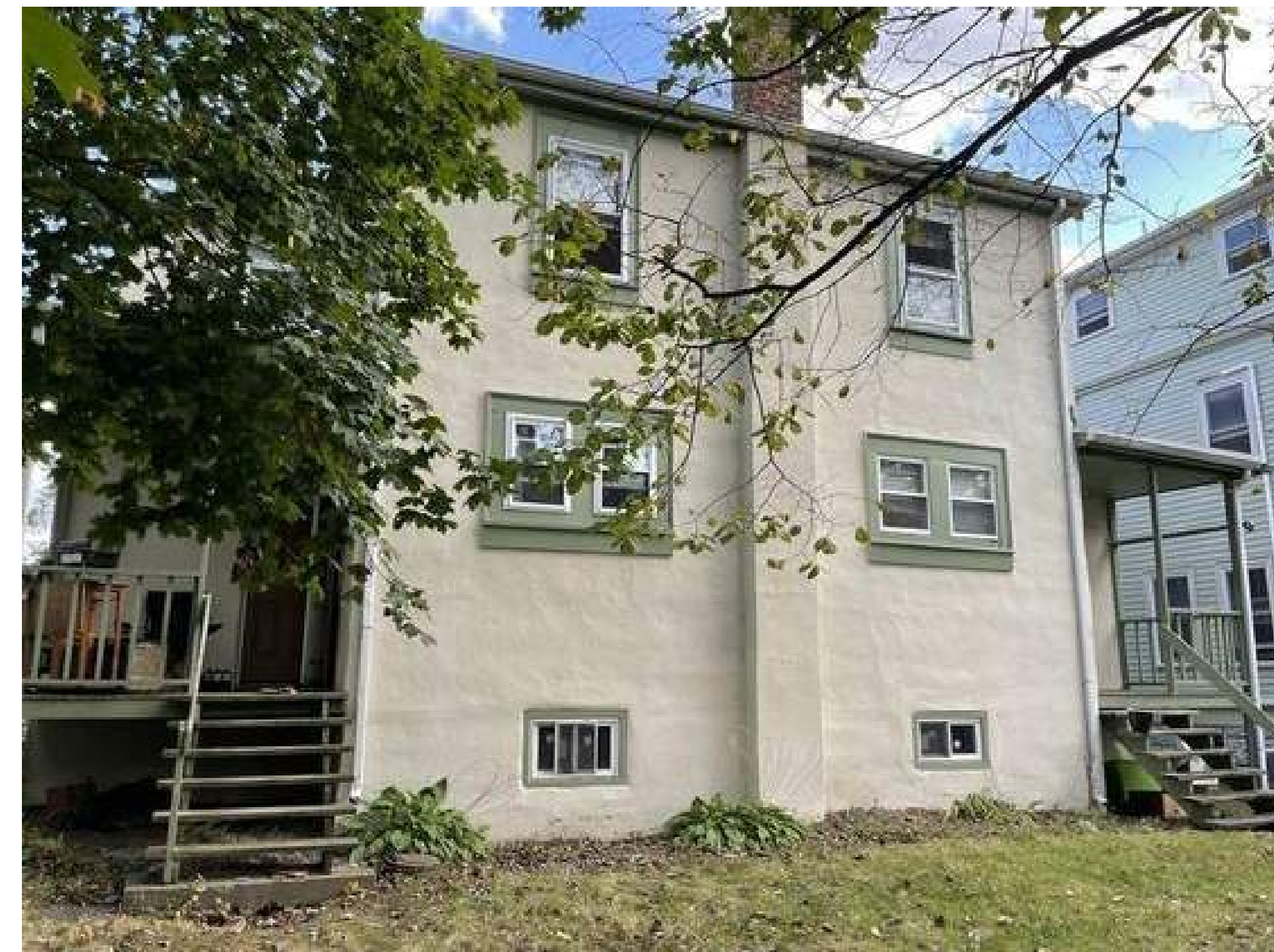
VIEW OF REAR
