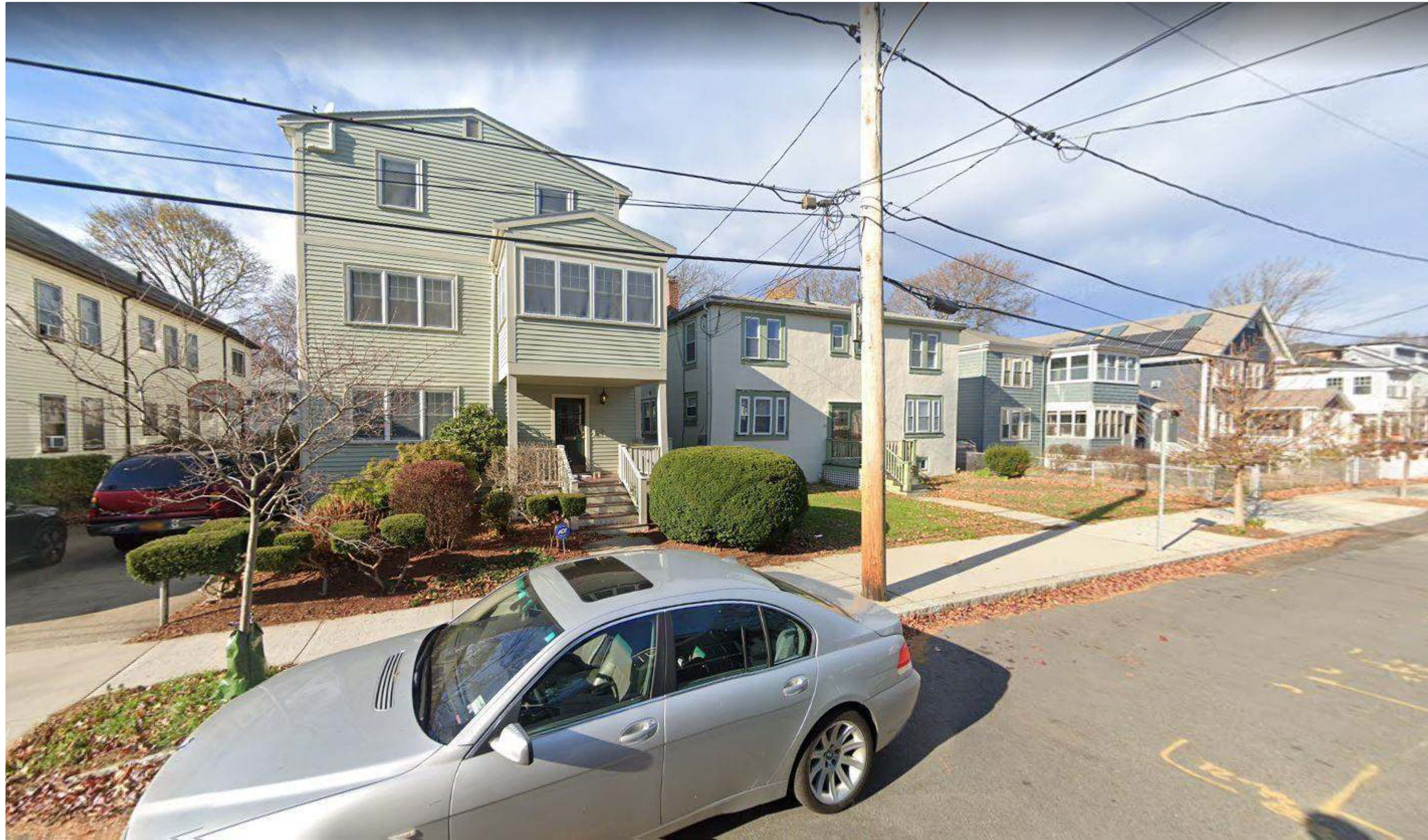
EXISTING STREET VIEW 2
