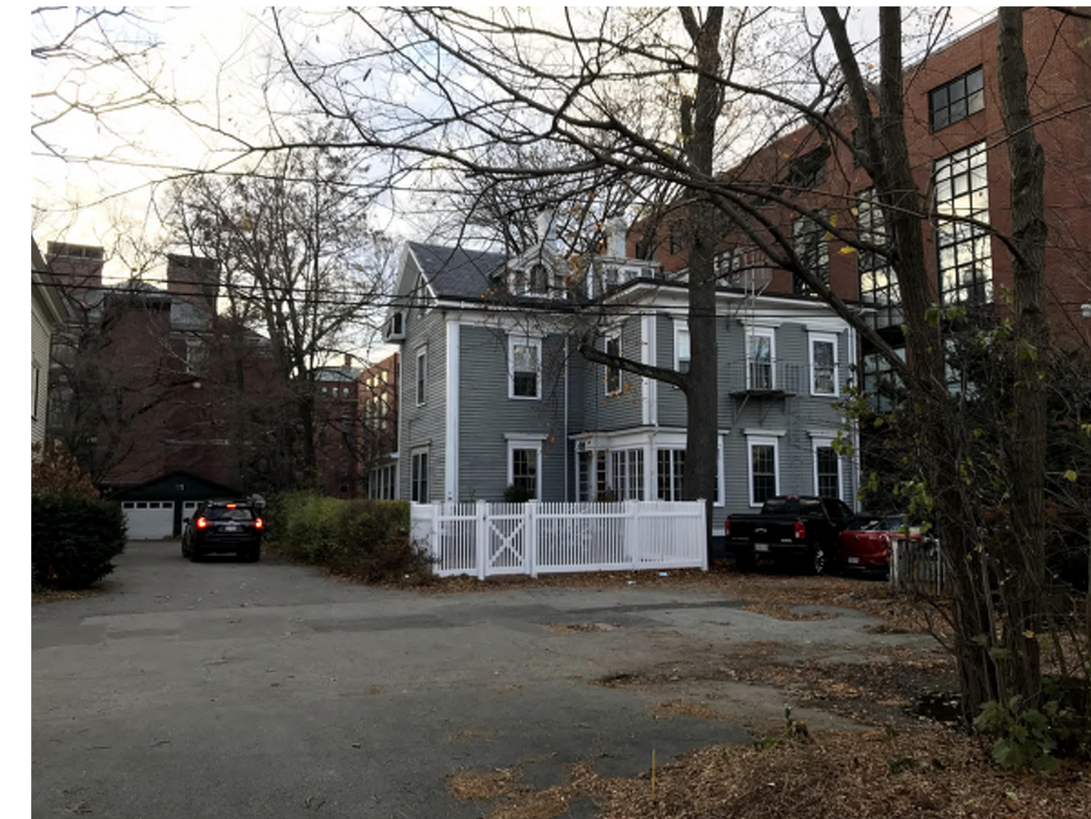
FRONT VIEW OF 13 KIRKLAND PLACE
