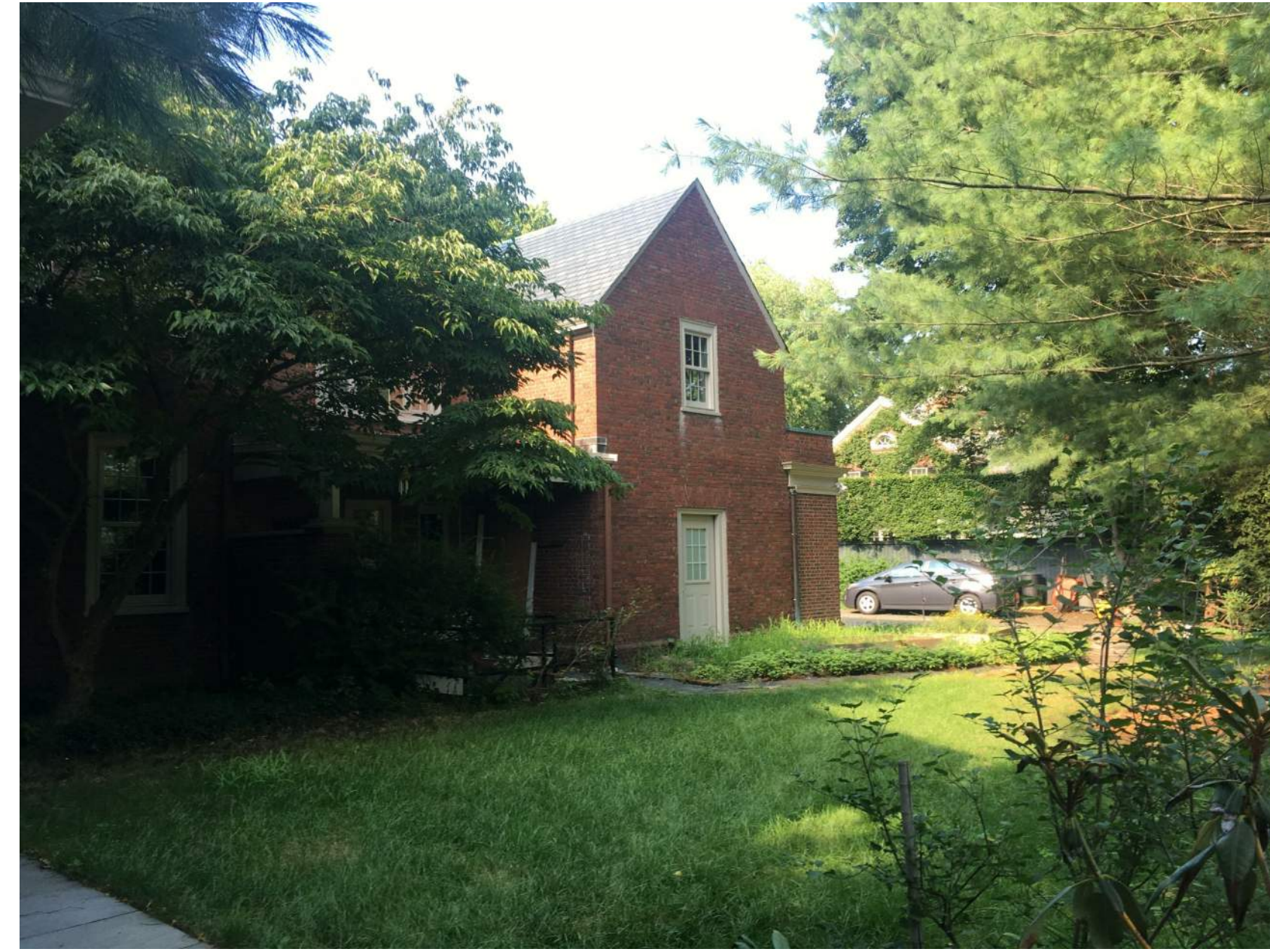
EXISTING SOUTH GARAGE VIEW
