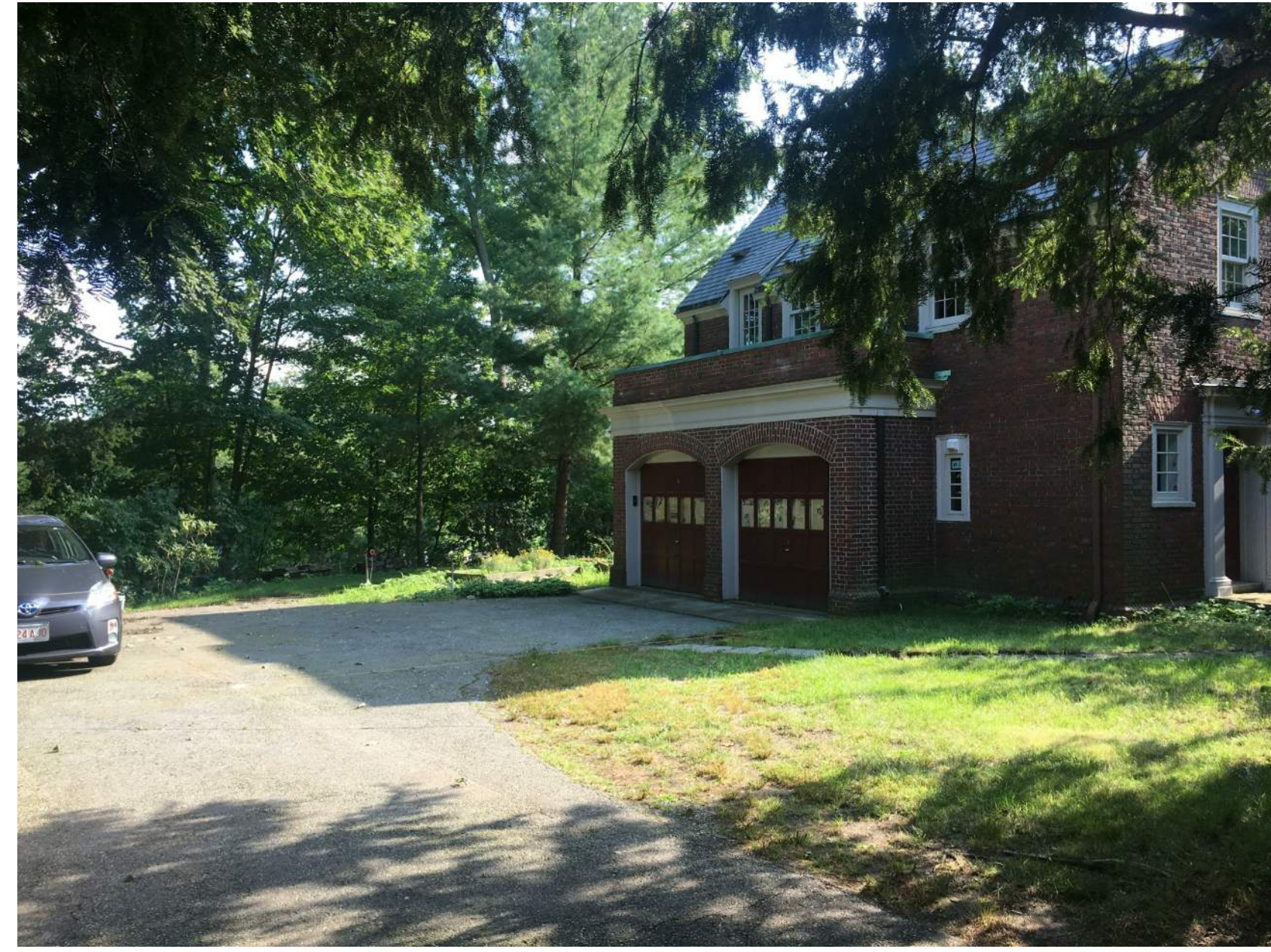
EXISTING NORTHEAST GARAGE VIEW
