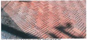
'PLANK' STYLE BRICK PAVER (PERMEABLE)
