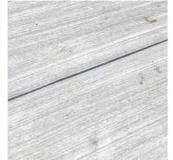
3 CITY STANDARD CONCRETE (SIDEWALK/ROW)
