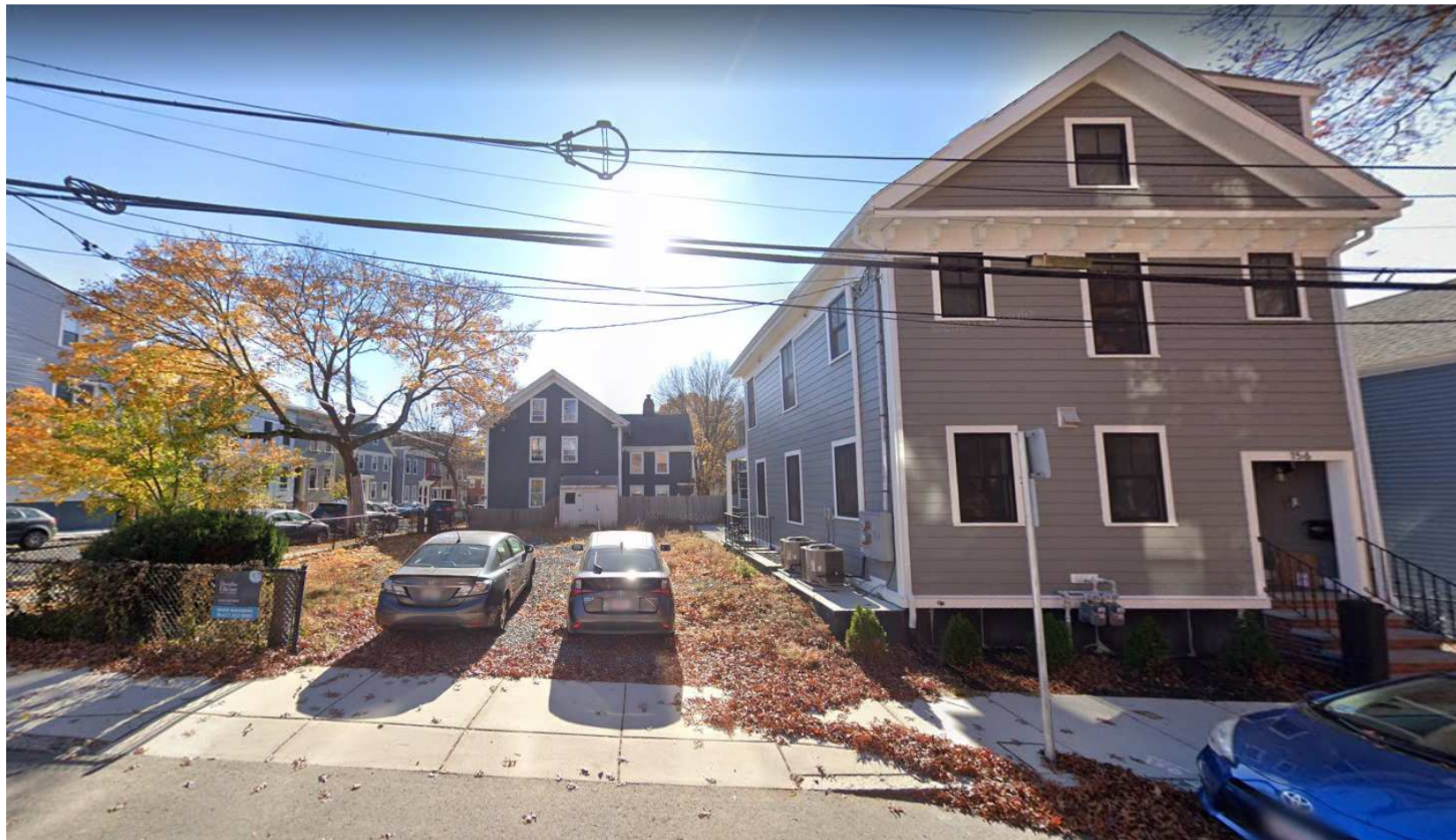
PRIOR TO ADDING 154 THORNDIKE RESIDENCE
