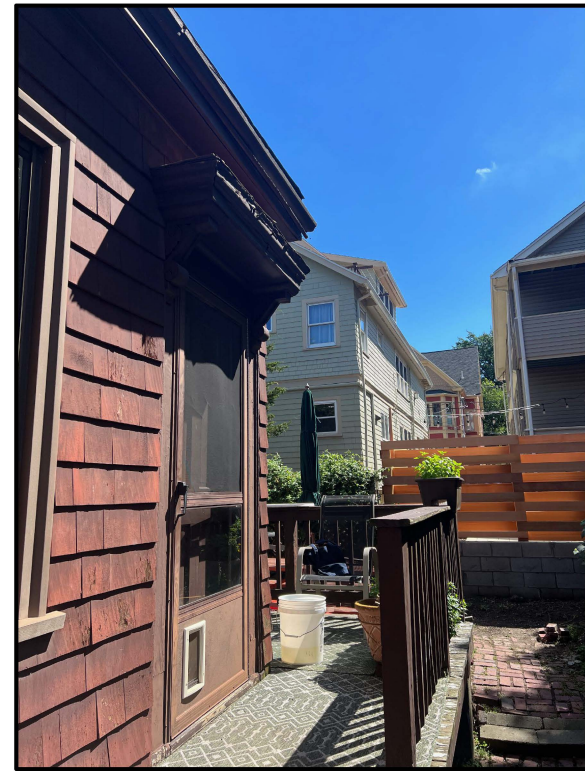
SIDE YARD VIEW OF BACK ENTRY & DECK
