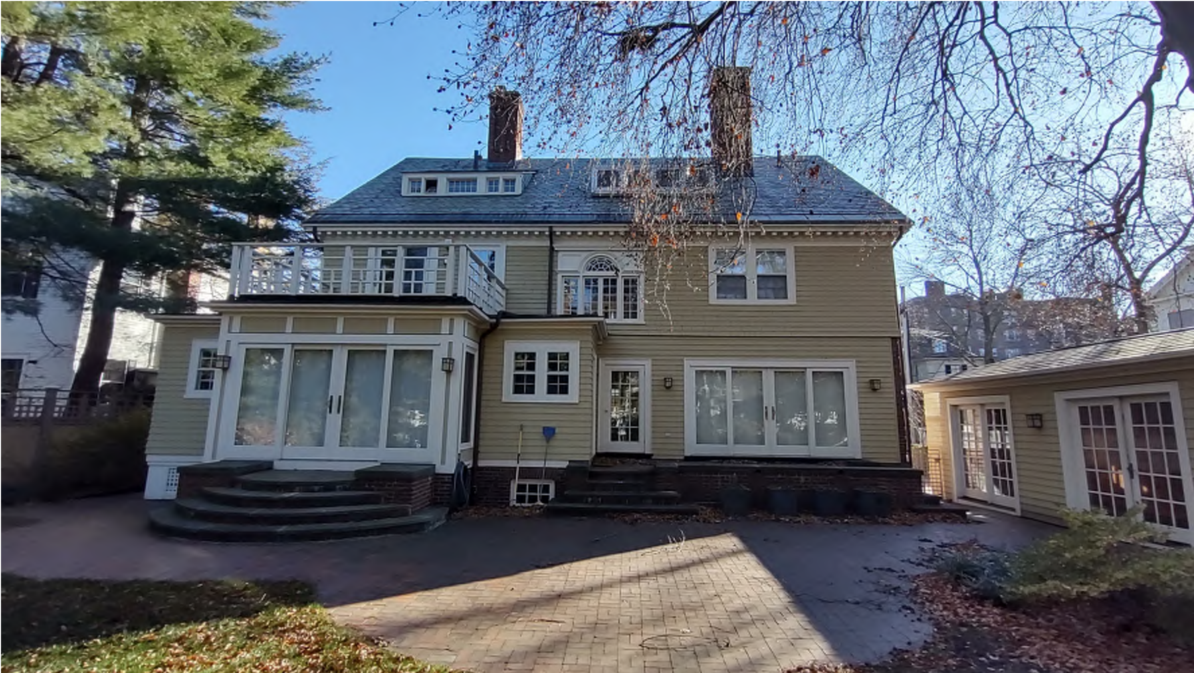
15 FOLLEN - BACK YARD FACADE (REAR)
