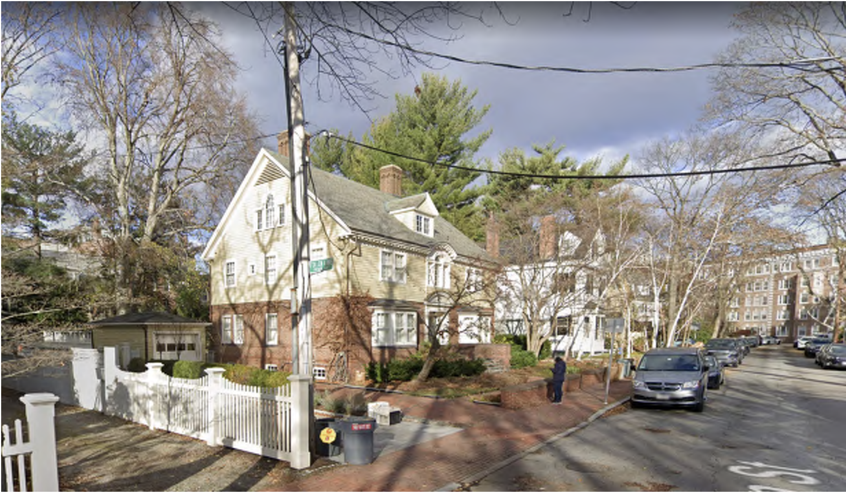
15 FOLLEN - VIEW FROM STREET LOOKING RIGHT
