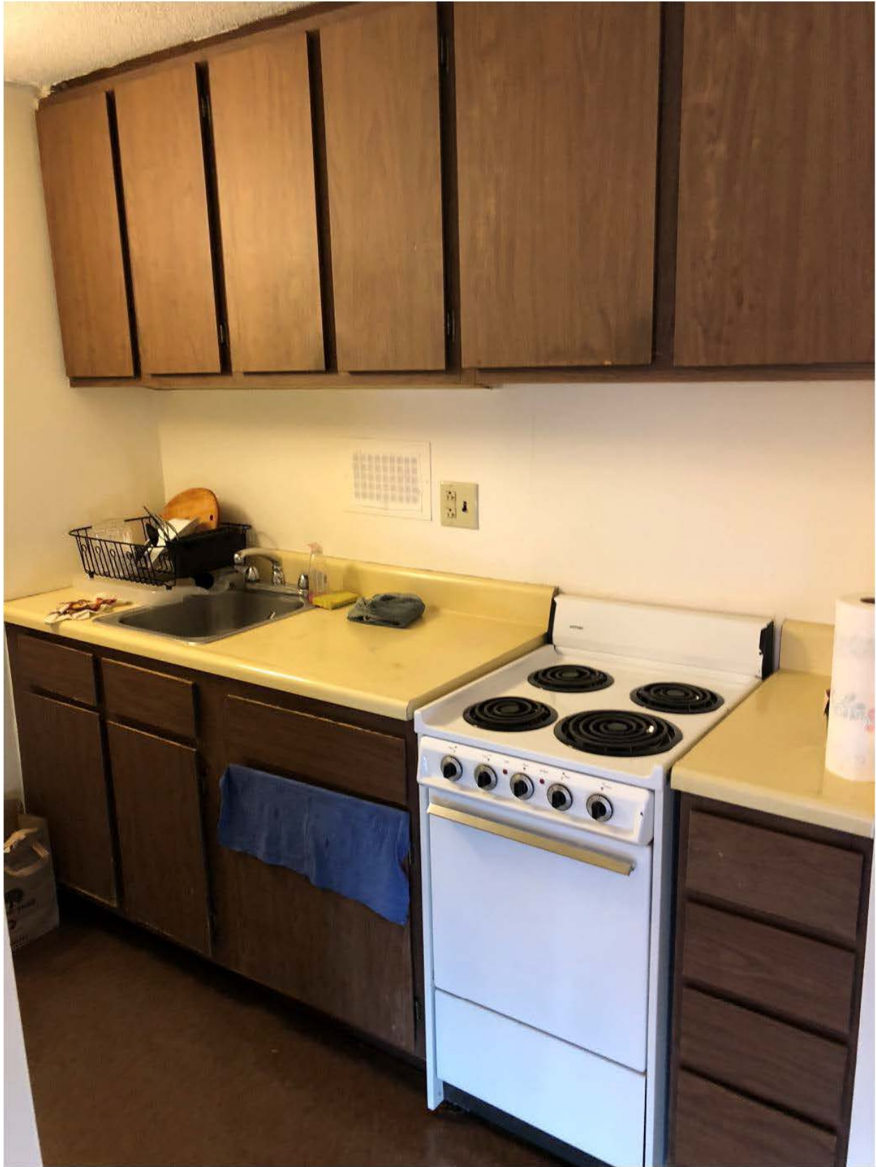
Interior Conditions 4 Typical Unit Kitchen
