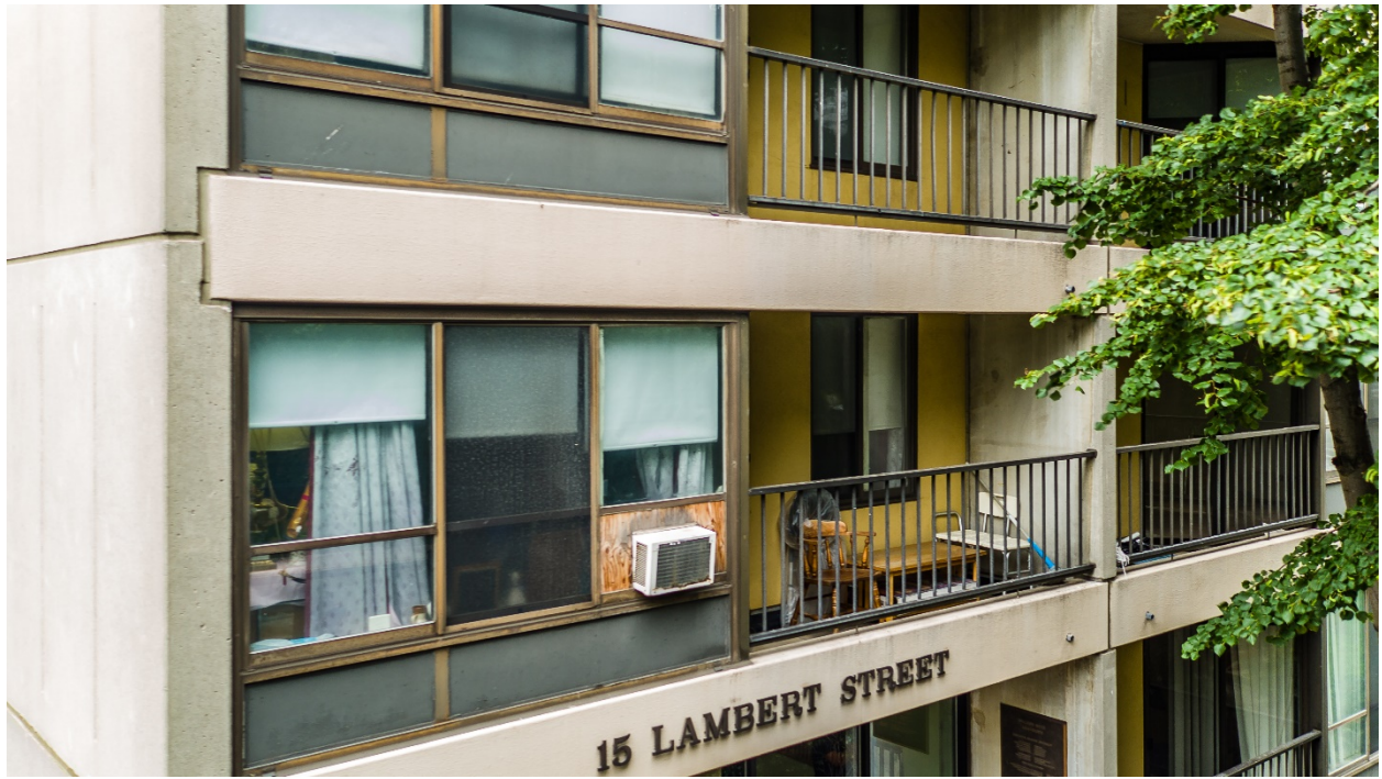
Exterior Condition 2 Lower Unit and Balconies
