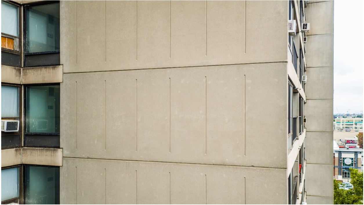
Exterior Condition 1 View along South face
