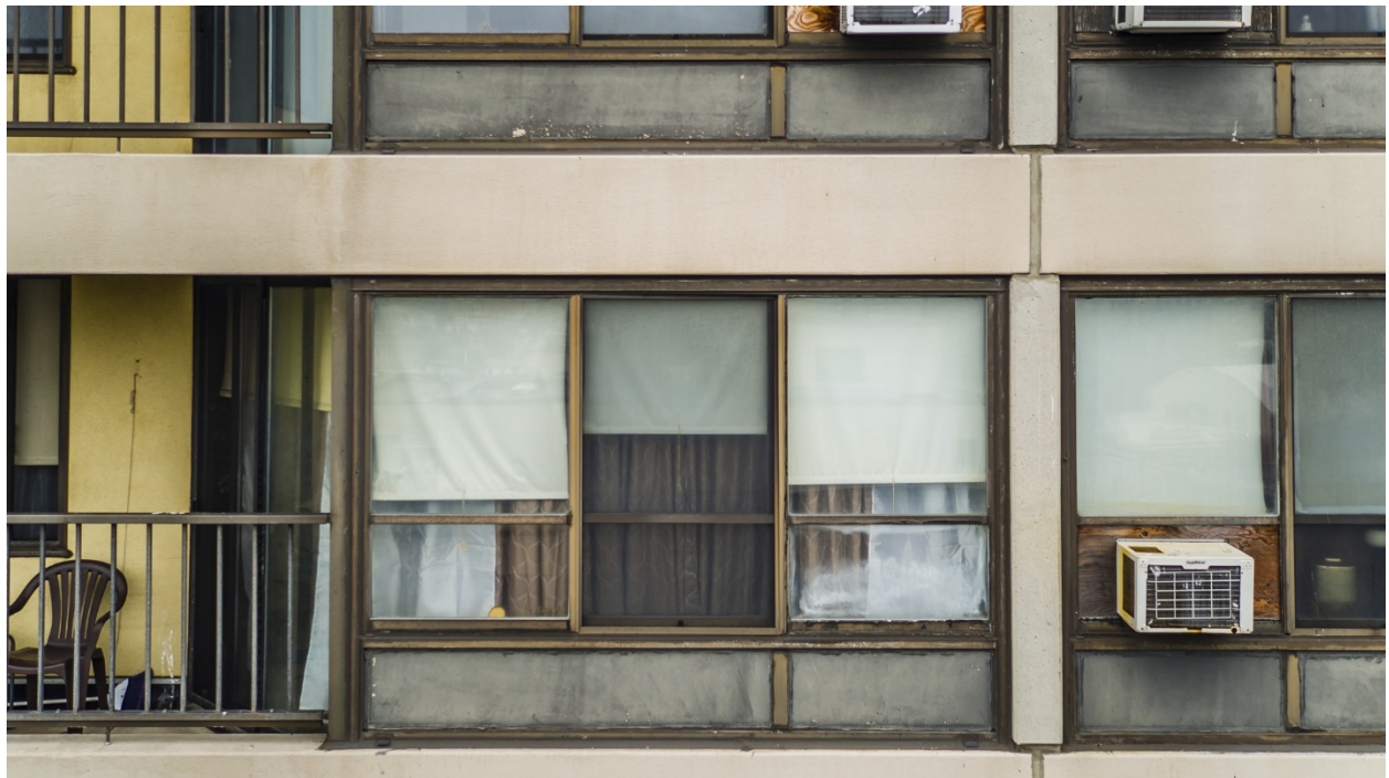
Exterior Condition 3 Upper Units and Balconies
