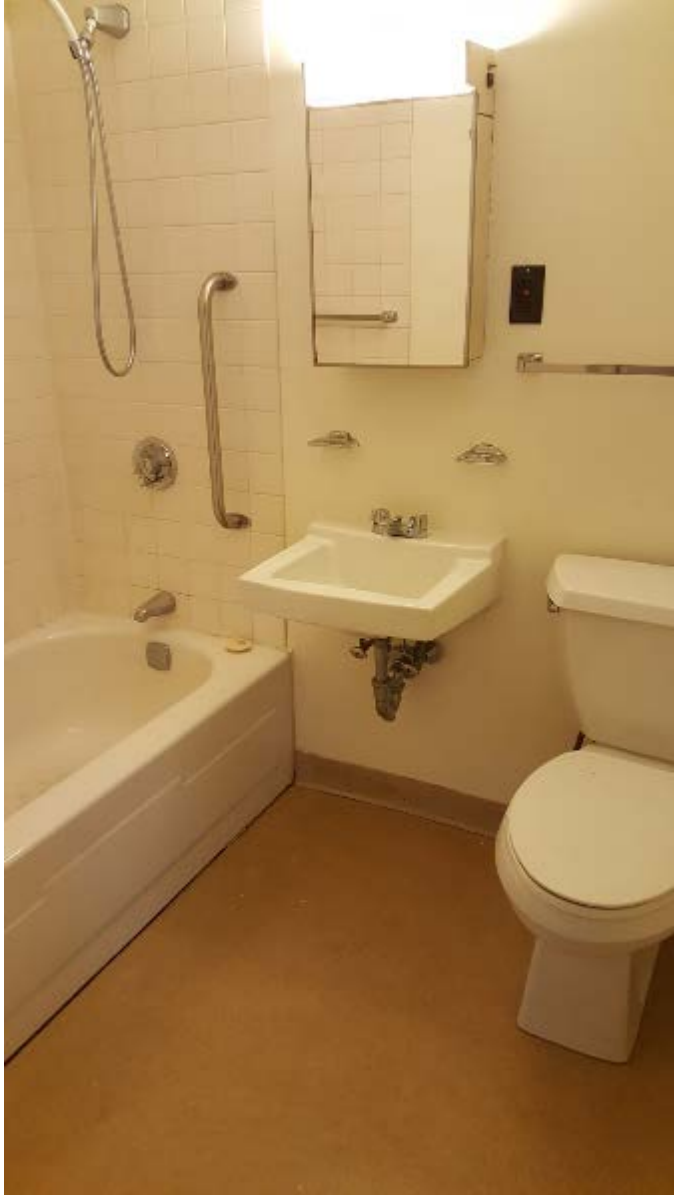
Interior Conditions 5 Typical Unit Bathroom
