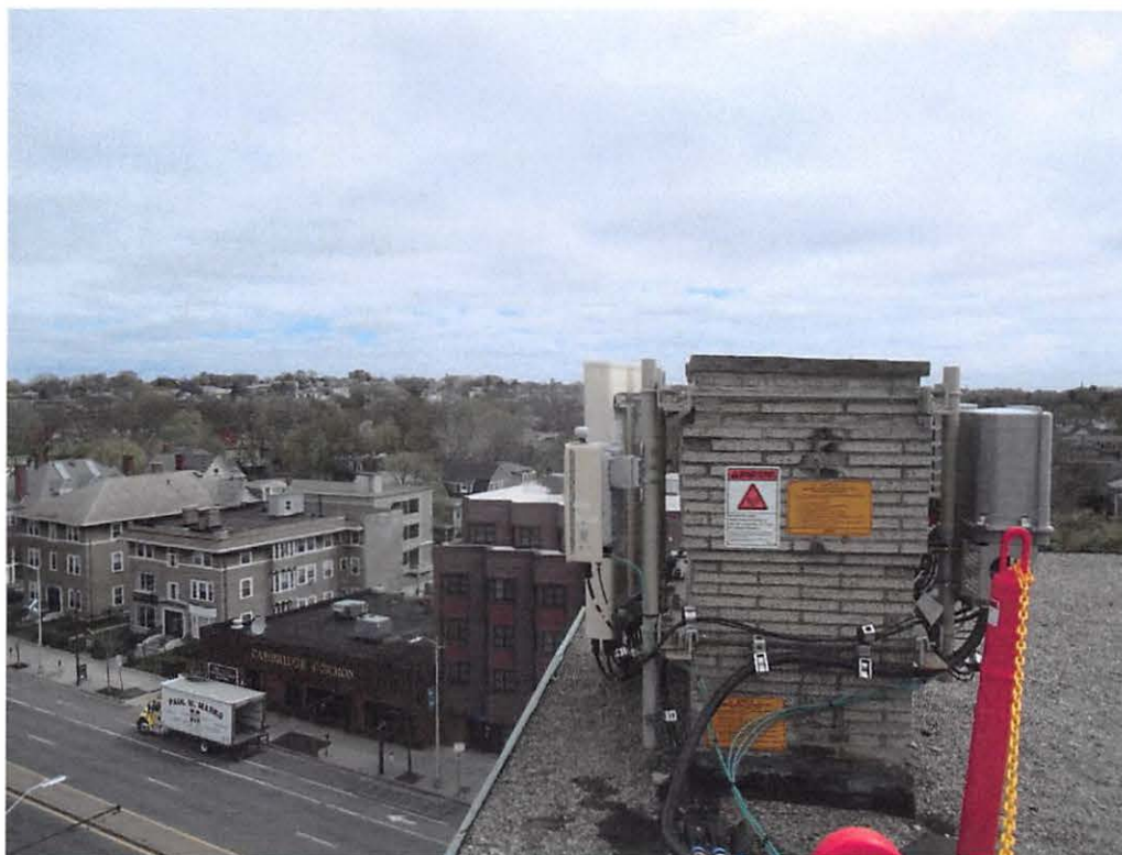
Exhibit A Existing Rooftop Photo
