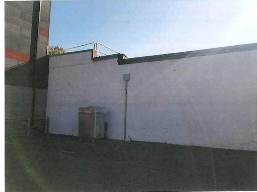
3. VIEW OF REAR SIDE OF STRUCTURE (FROM PARKING LOT)
