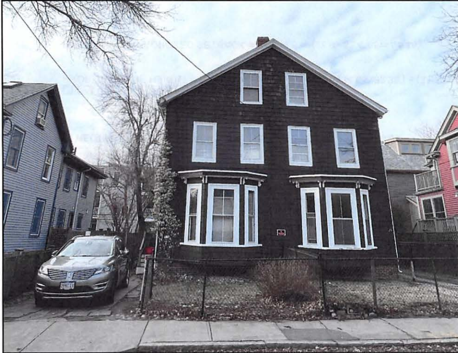
EXISTING STREET VIEW
