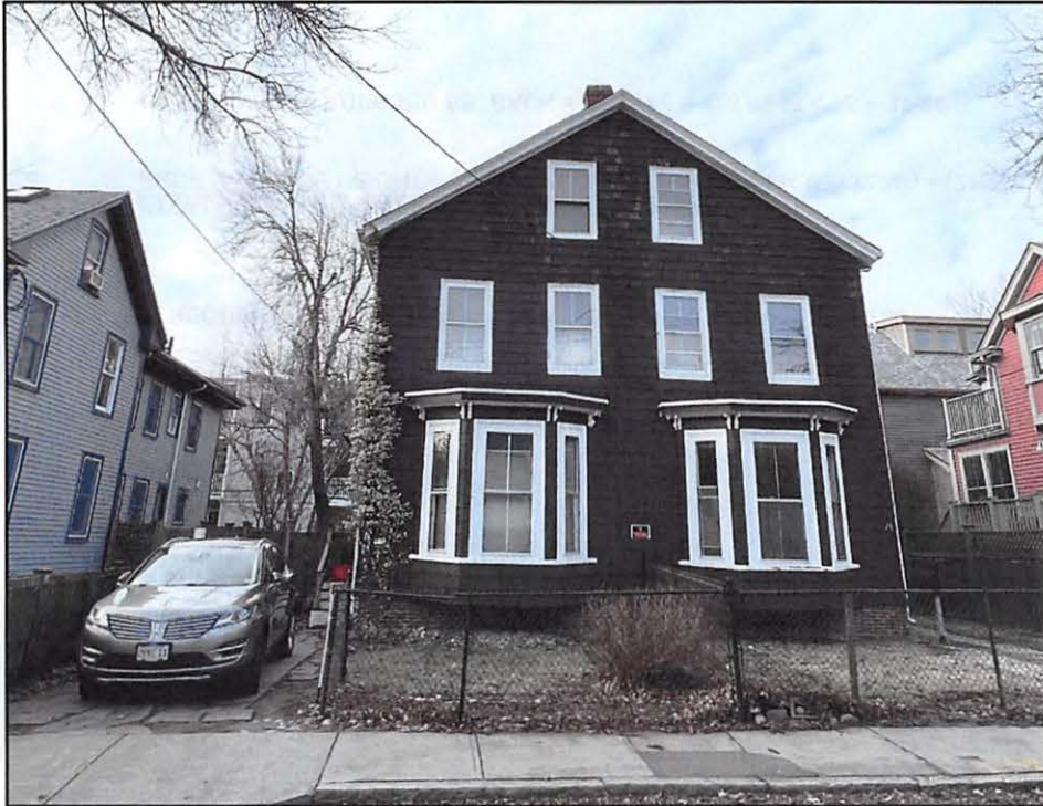
EXISTING STREET VIEW
