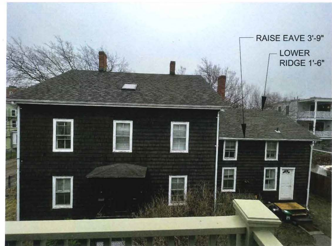
VIEW FROM 22 FAIRMONT ST 2ND FLOOR DECK
