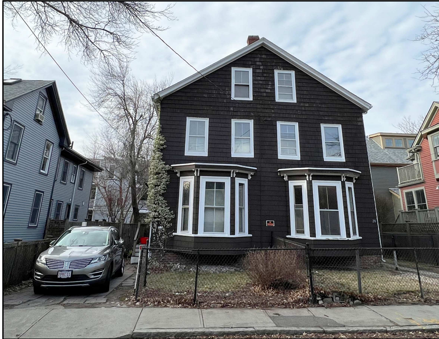
EXISTING STREET VIEW
