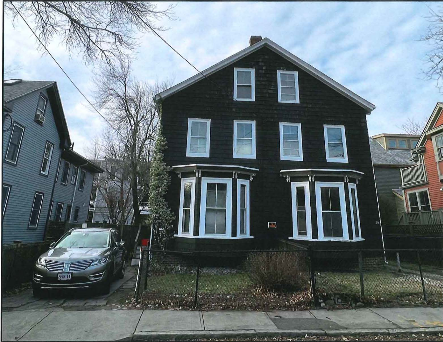
EXISTING STREET VIEW
