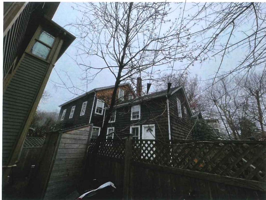
VIEW OF REAR BUMPOUT FROM YARD OF 24 FAIRMONT STREET
