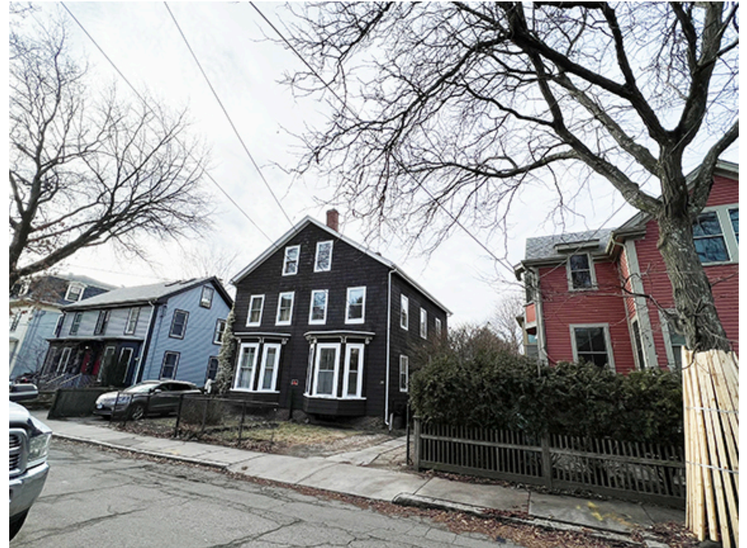
STREET VIEW 18-20 FAIRMONT STREET
