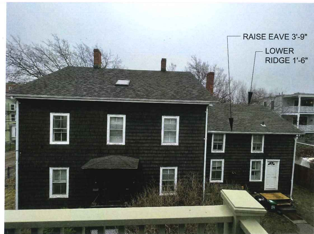
VIEW FROM 22 FAIRMONT ST 2ND FLOOR DECK
