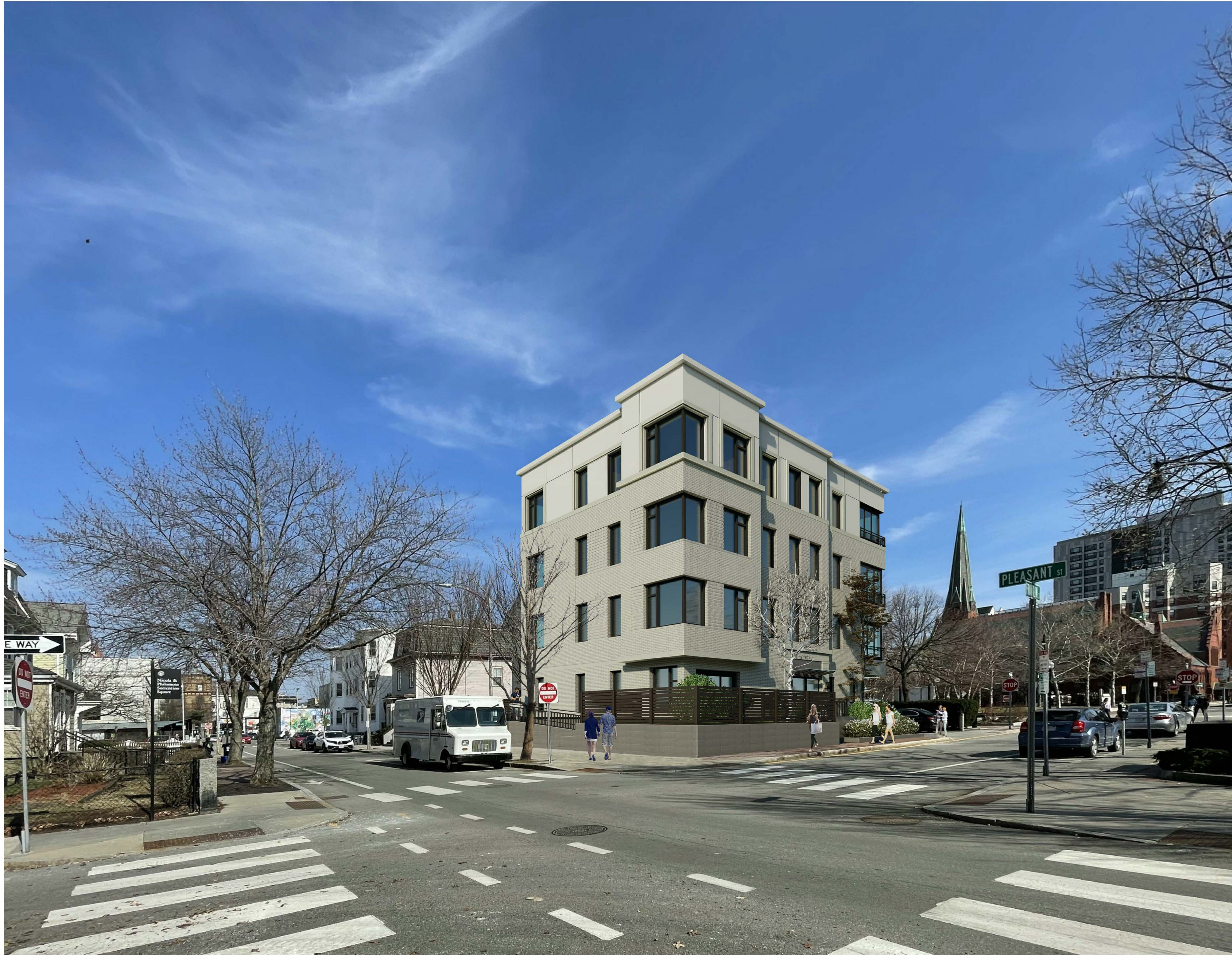
VIEW AT PLEASANT ST & FRANKLIN ST
