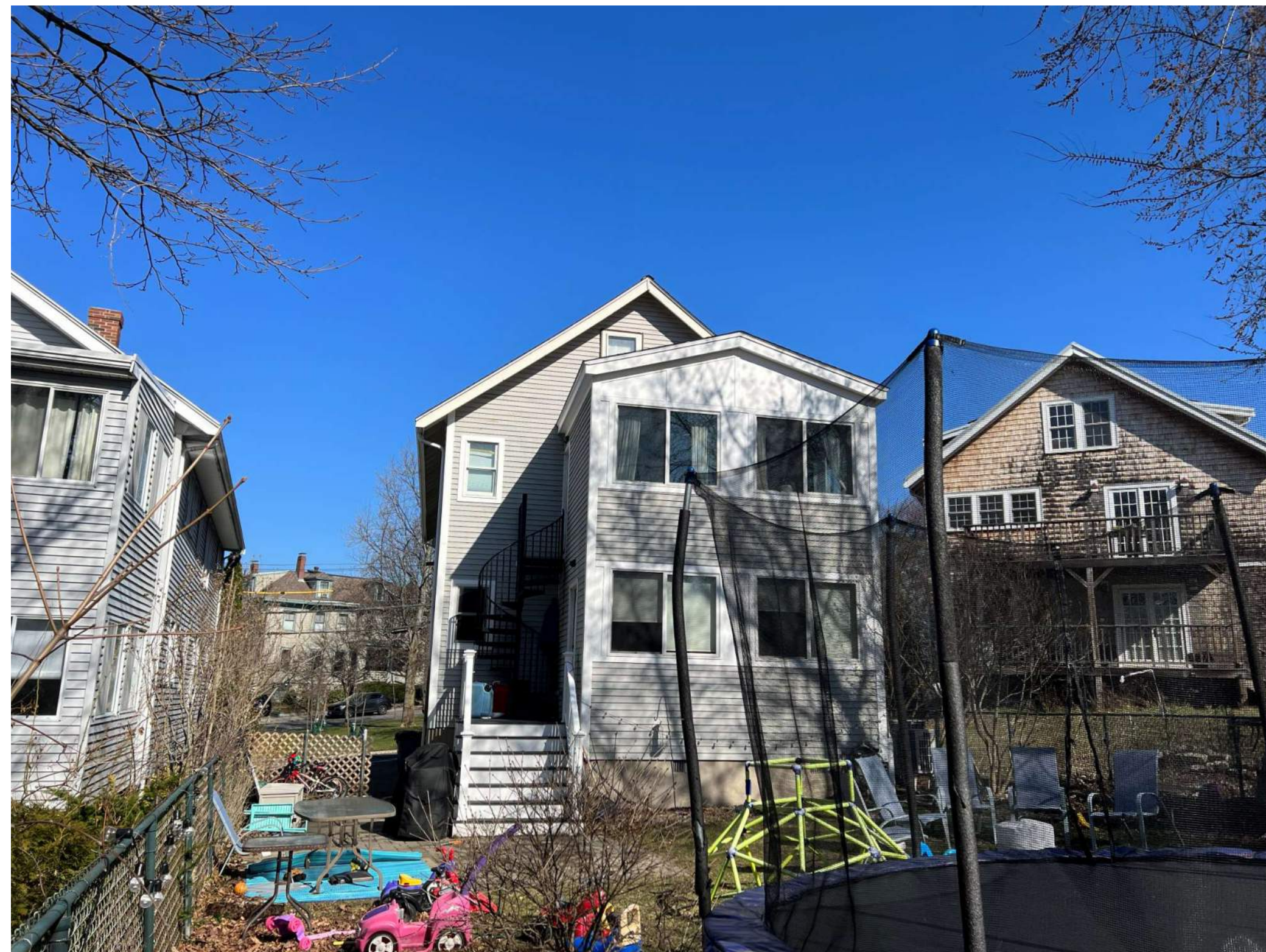
EXISTING VIEW OF REAR & RIGHT ELEVATIONS FROM REAR YARD
