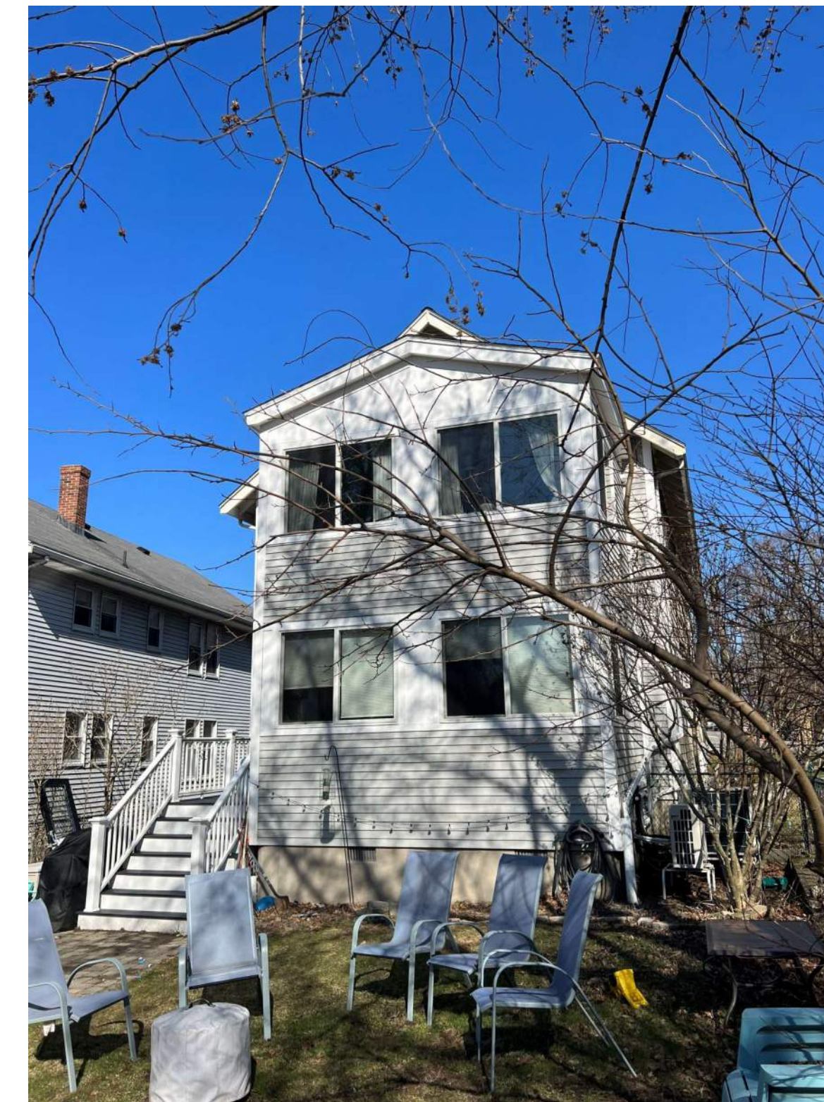
EXISTING VIEW OF REAR & LEFT ELEVATIONS FROM REAR YARD
