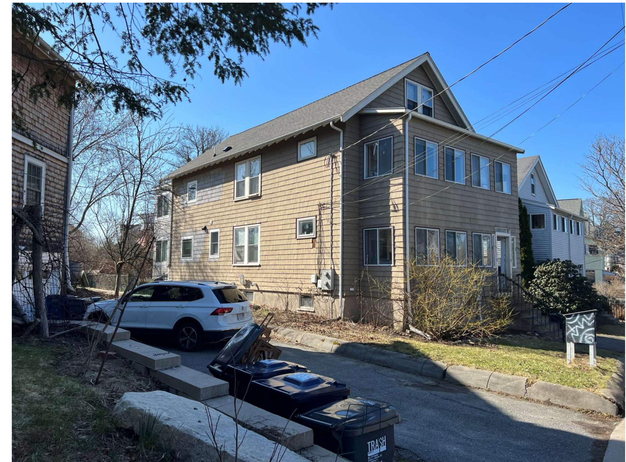
EXISTING VIEW OF FRONT & LEFT ELEVATIONS FROM FOUNTAIN TERRACE
