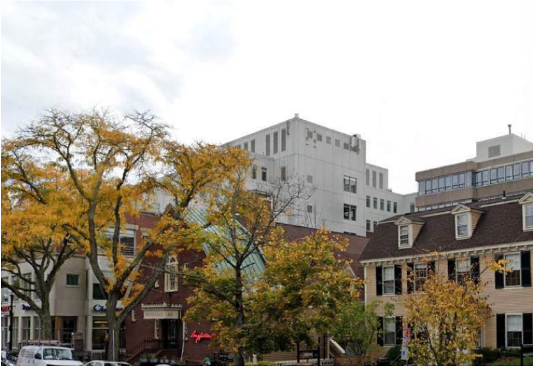
3. View of the host structure facing south from Church Street within the Harvard Square Historic District (Boundary Expansion).
