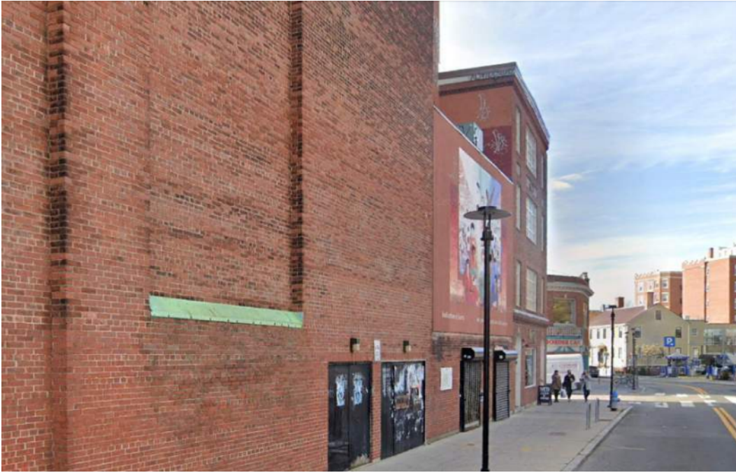
9. View from the Cambridge Common Historic District facing southwest towards the host structure along Church Street.
