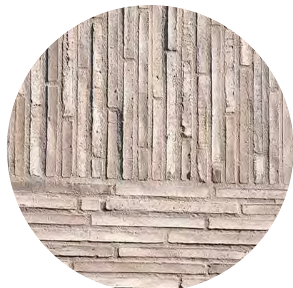
MASONRY SOLDIER COURSE AT HEADER
