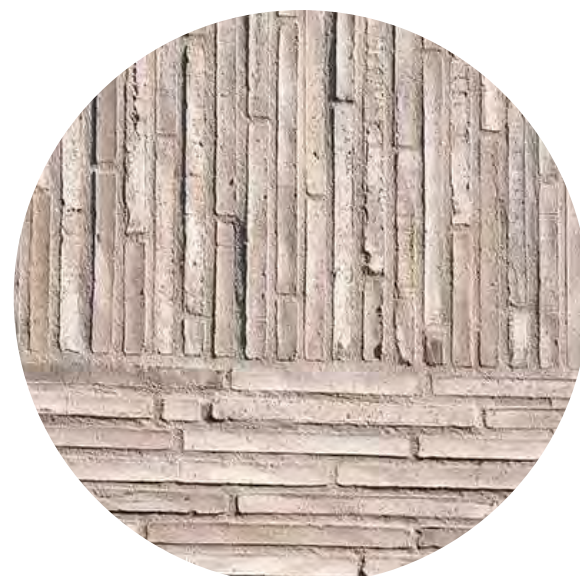
MASONRY SOLDIER COURSE AT HEADER
