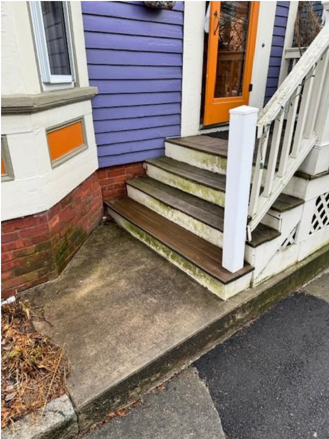
Figure 2: 20 Fairmont Ave, Existing concrete step to be removed
