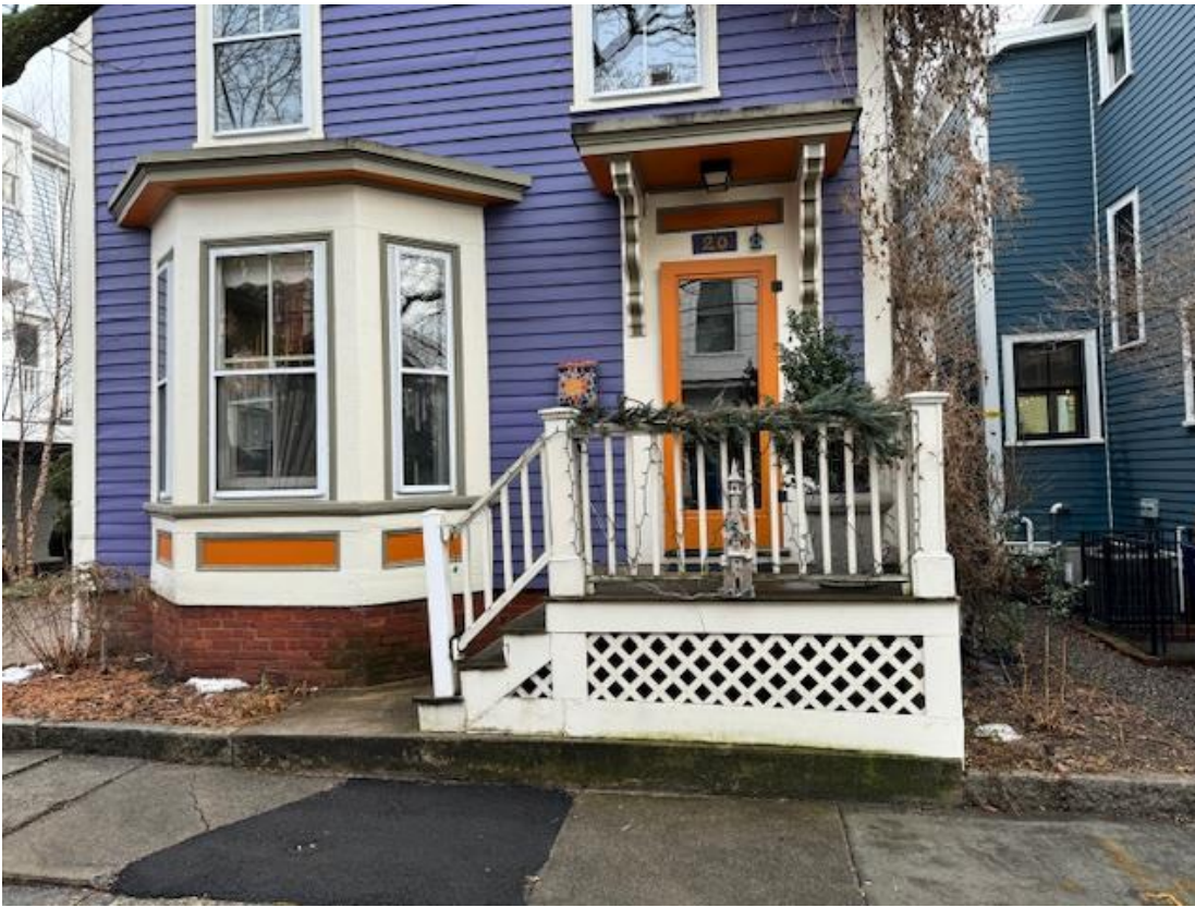
Figure 1: 20 Fairmont Ave Existing Porch
