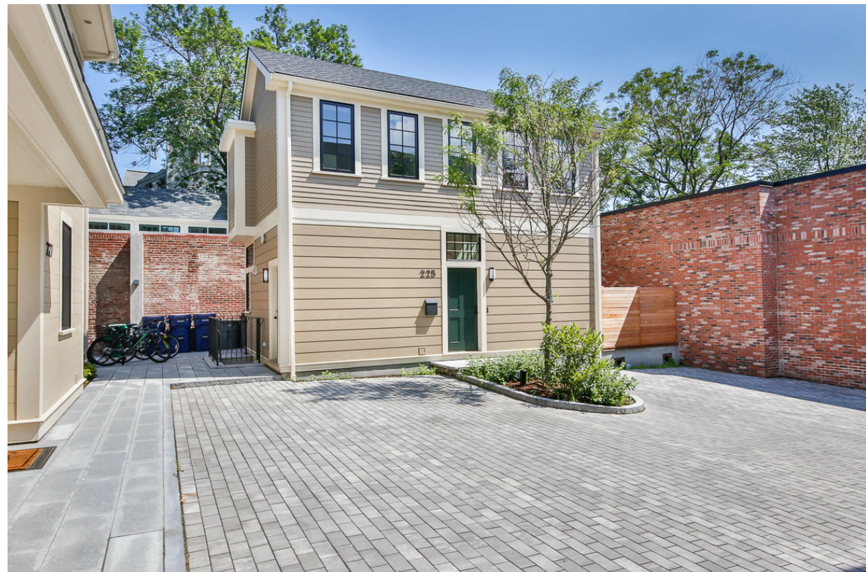
225 CONCORD AVE (CENTER), 227 CONCORD AVE (LEFT), 221-223 CONCORD AVE (RIGHT)
