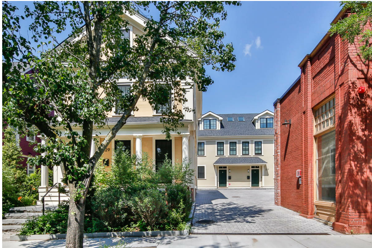
229 CONCORD AVE (LEFT), 227 CONCORD AVE (CENTER), 221-223 CONCORD AVE (RIGHT)
