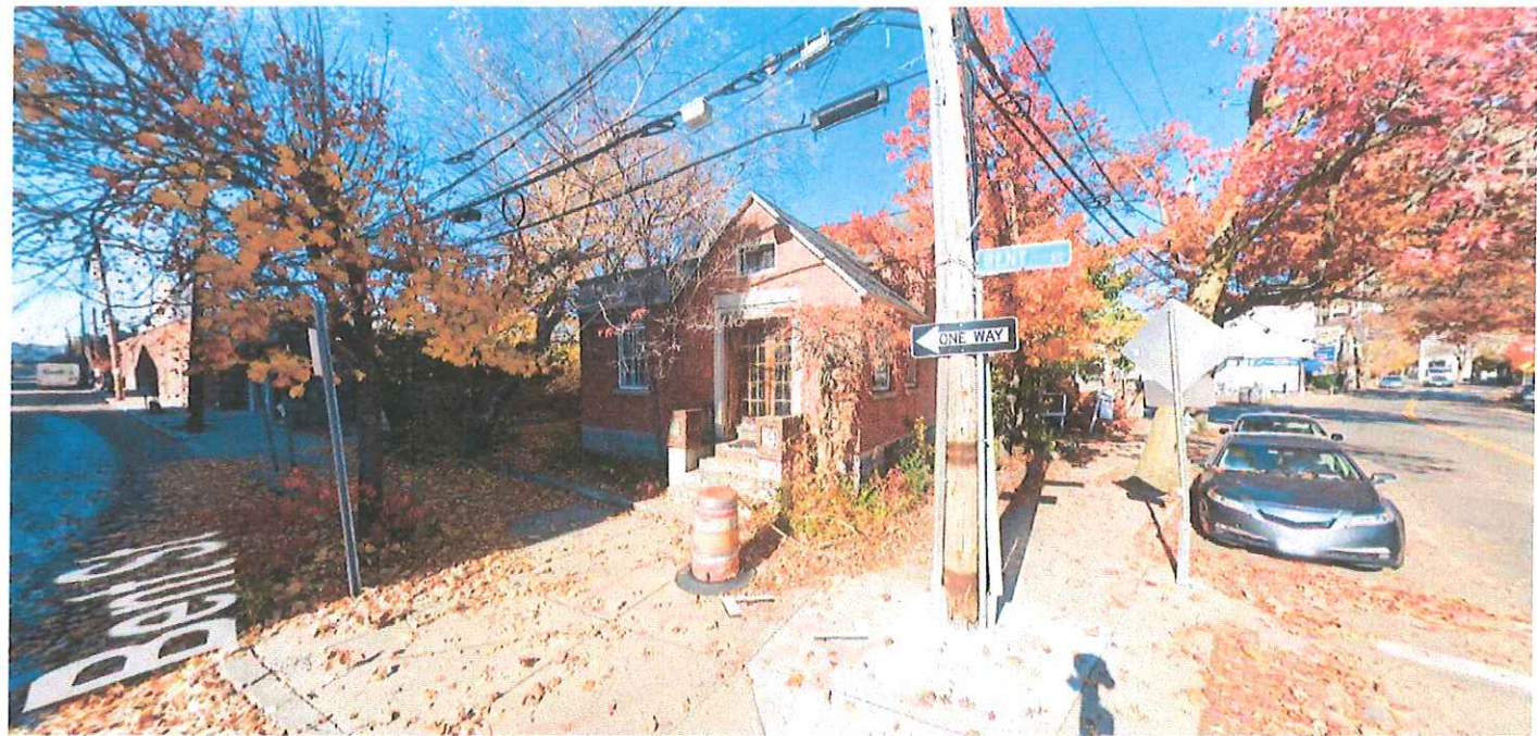
235 THIRD STREET AT CORNER OF BENT
