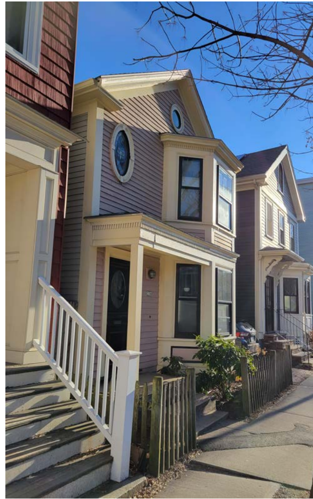
FRONT FACADE PROSPECT STREET VIEW
