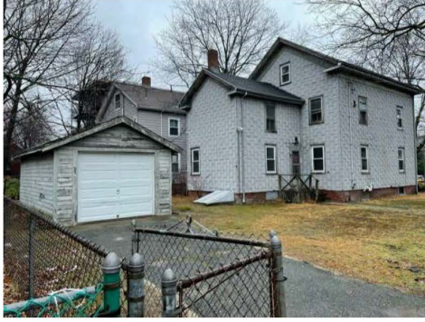
VIEW FROM ALLSTON STREET
