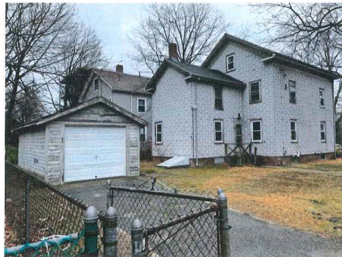
VIEW FROM ALLSTON STREET
