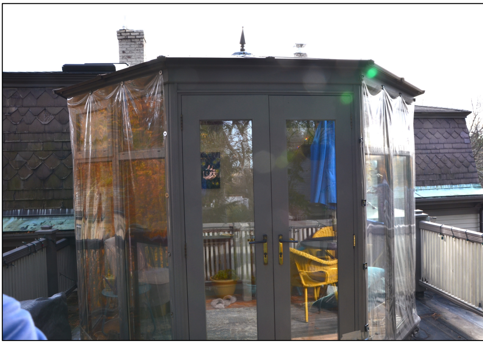
On 3 rd floor deck looking at sunroom from the NNW
