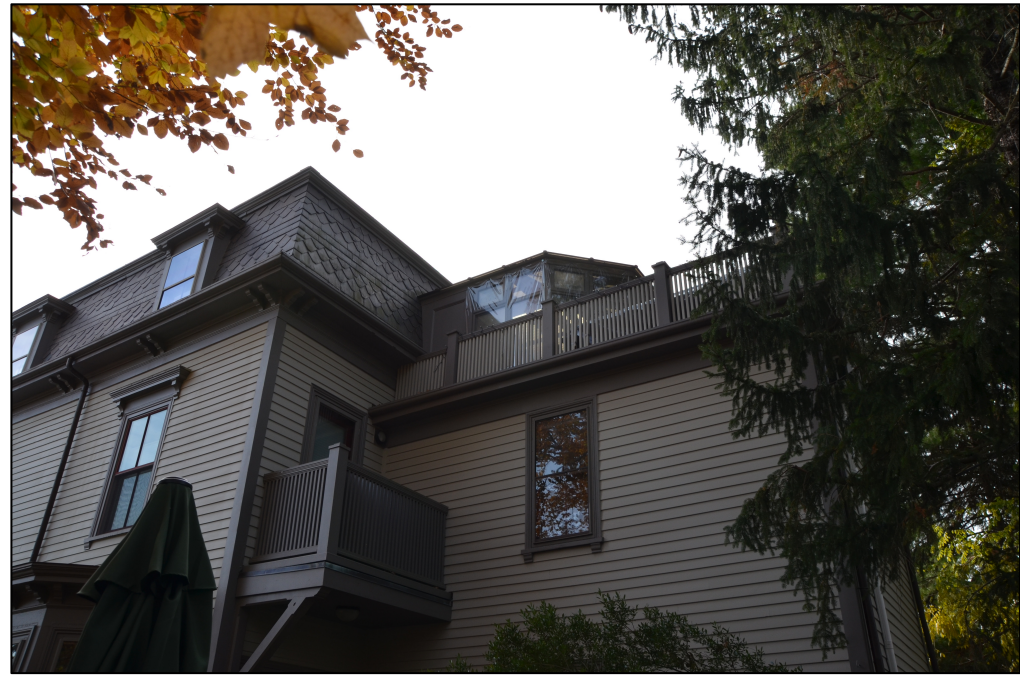
On the ground looking at sunroom from the northeast
