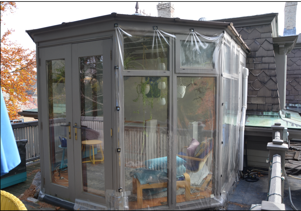
On 3 rd floor deck looking at sunroom from the northwest
