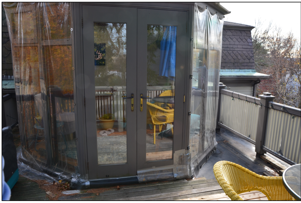
On 3 rd floor deck looking at sunroom from the NNW
