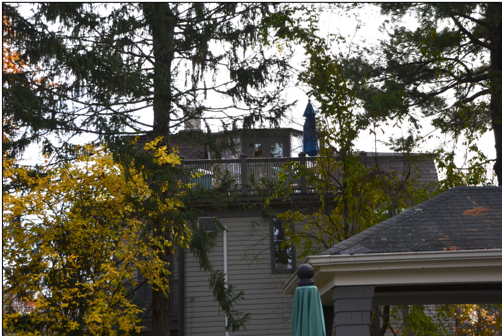
On the ground looking at sunroom from the NNW
