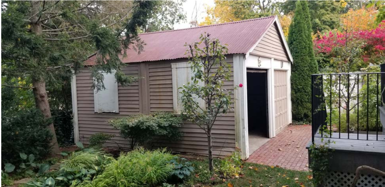
Existing Garage (west face); Boarded windows and damaged siding to be removed, structure to be reinforced, new openings to be added
