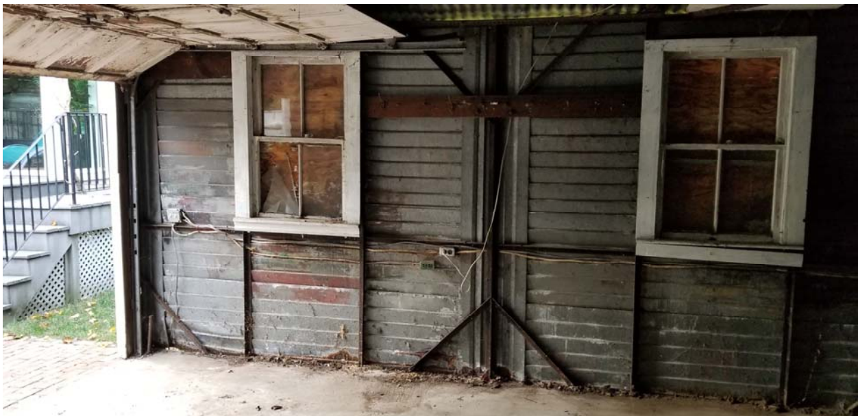
Existing Garage, interior (west side); Broken windows and damaged siding to be removed, structure to be reinforced, new openings to be added
