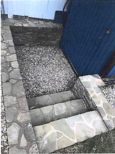
Stairwell to 14B Bellis Circle shed in dry conditions
